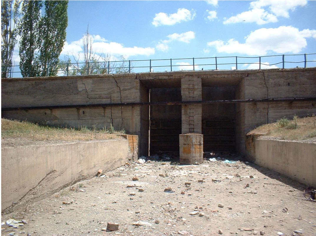
Figure 3.38 Water Control Structure of Lake Eymir (DSİ, 2008)
