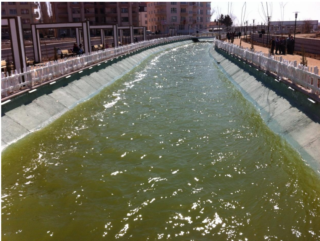
Figure 3.31 General View of Lined Canal between Mogan and Eymir Lakes
