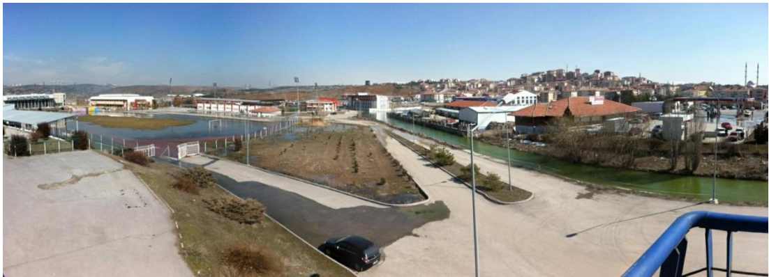
Figure 3.33 Flooding Areas at the Downstream of Lake Mogán (20.03.2012)
