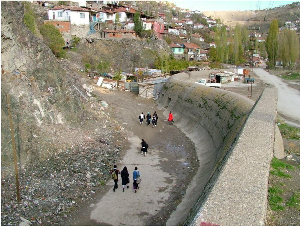
Figure 3.41 Spillway of İncesu Detention Pond (DSİ, 2008)
