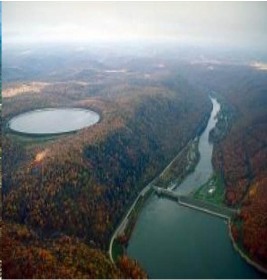
Figure 3.2b Kinzua Dam and PSHP (Pennsylvania, USA)
