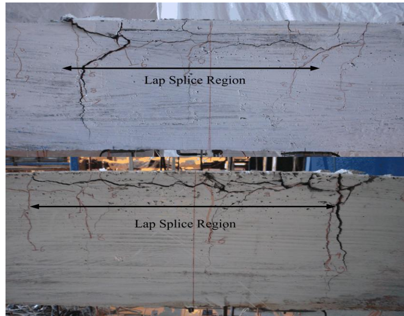
Figure 4.30 Cracks formation and side splitting occurrence on the side cover of the specimen
