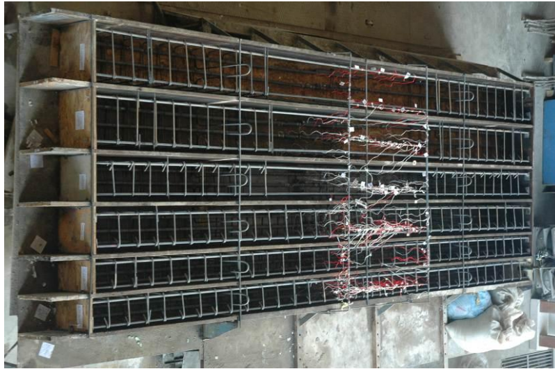
Figure 3.5 Formwork with reinforcement cage
