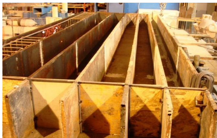
Figure 3.4 Finished view of formwork
