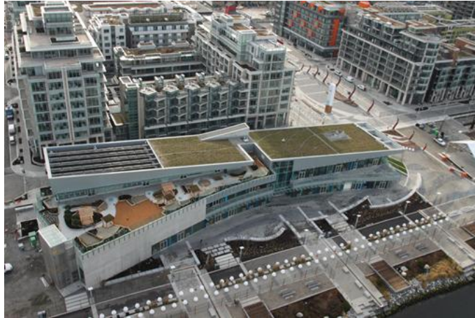
Figure 27: Green roof of the community centre and the solar collectors next to it ( www.milkovicharchitects.com )
