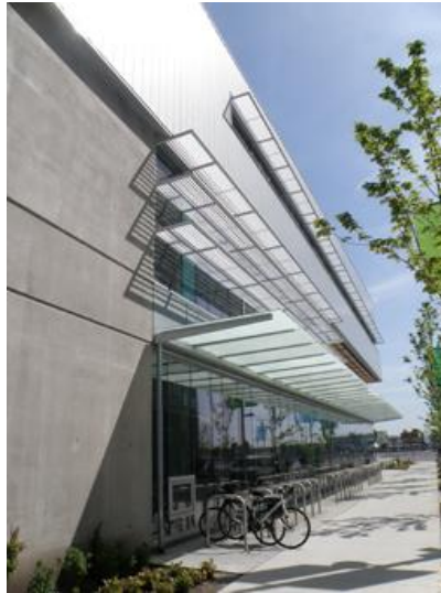
Figure 30: Openings in the facade of the centre (milkovicharchitects.com)
