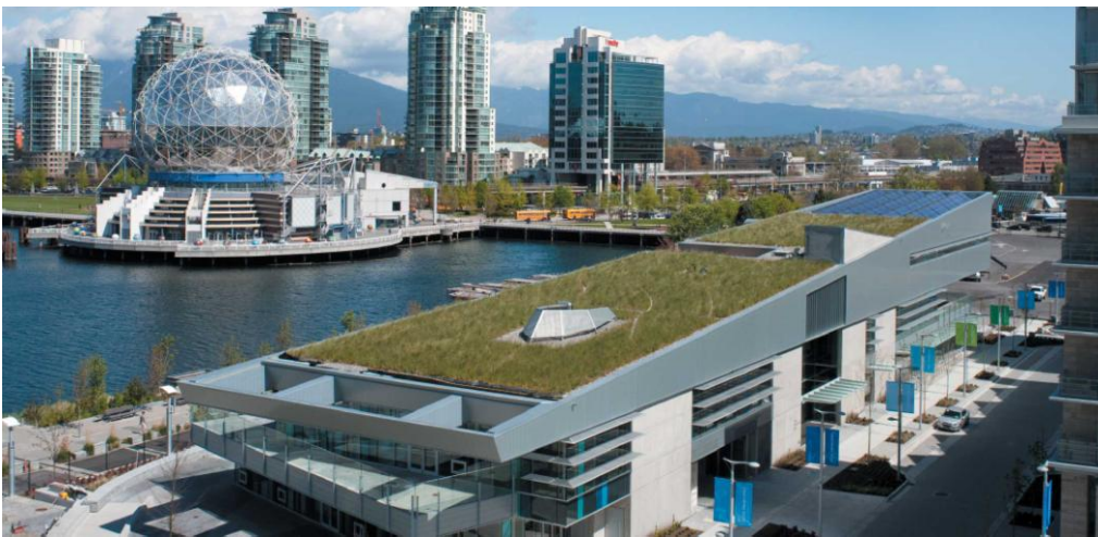
Figure 25: Creekside Community Centre in waterfront of Vancouver (www.sabmagazine.com)
