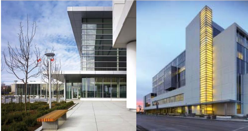
Figure 35: Views of the courthouse (www.canadianarchitect.com)
