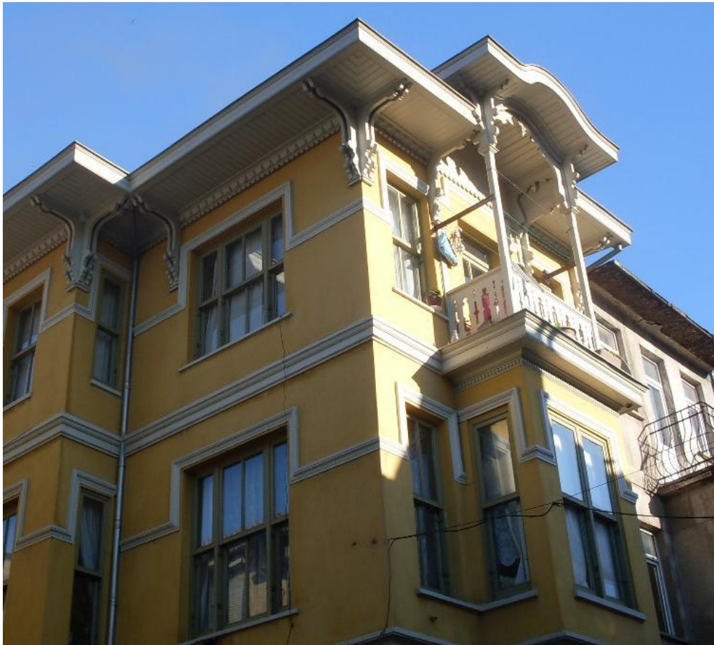
Figure 65: Projection and balcony of Building on Block 2307 Lot 28 after the restoration
