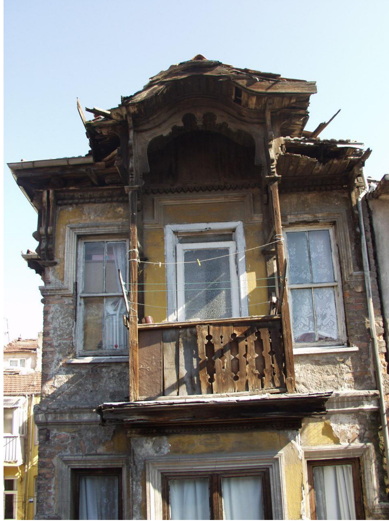
Figure 62: Balcony of Building on Block 2307 Lot 28 before the restoration (Altınsay Özgüner, 2009)
