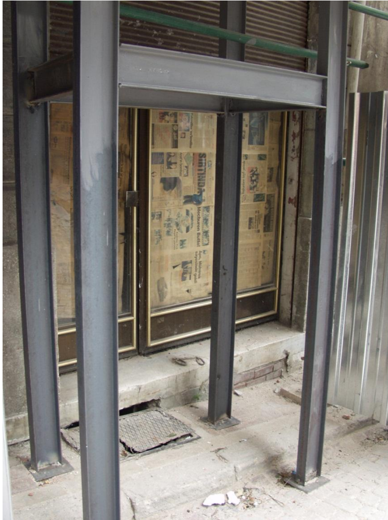
Figure 120: Restoration implementations in FBDRP (Altınsay Özgüner, 2009)
