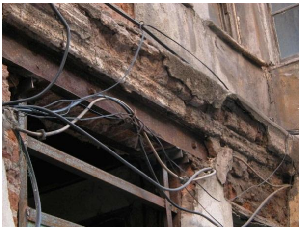
Figure 59: Condition of Fener Balat houses (Altınsay Özgüner, 2009)
