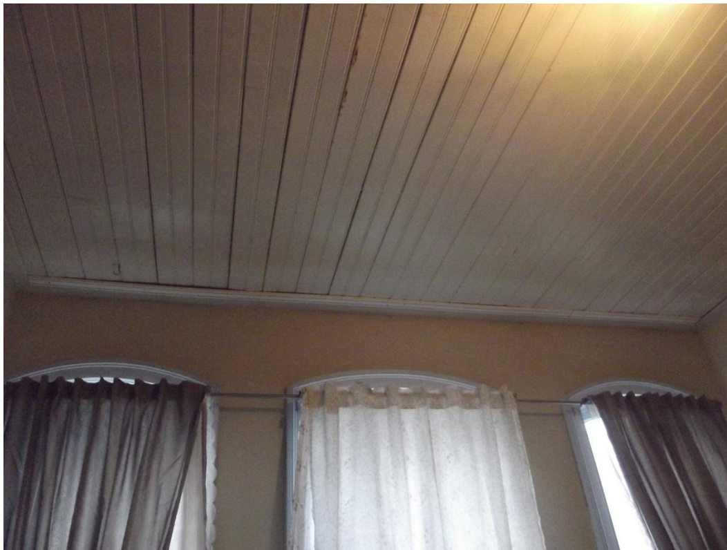
Figure 70: Ceiling of first floor after the restoration
