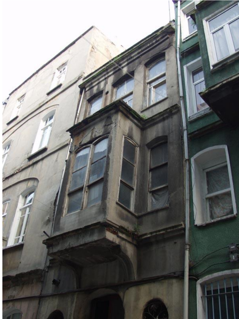
Figure 68: Building on Block 2307 Lot 28 before the restoration ( www.fenerbalat.org )
