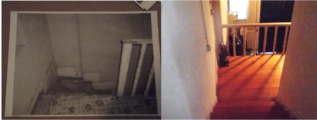
Figure 69: Staircases before and after the restoration (old photo found in the house)
