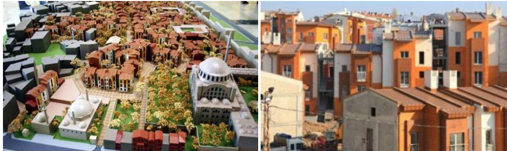
Figure 1: Model for Sulukule Renewal Project ( www.emlakrotasi.com ) and Sulukule after the Project ( www.konuthaberleri.com )
