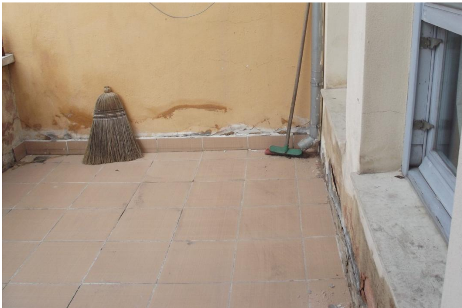
Figure 74: New ceramic floor tiling and skirting
