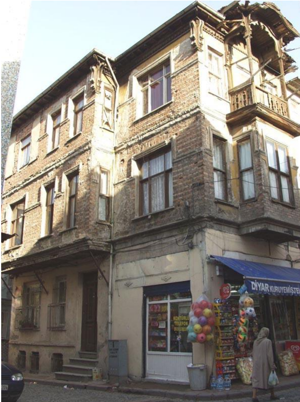
Figure 61: Building on Block 2307 Lot 28 before the restoration ( www.fenerbalat.org )
