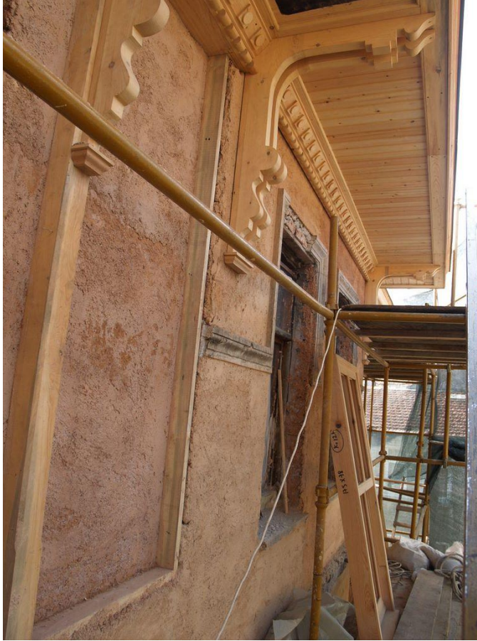
Figure 63: Roof repair of the building on Block 2307 Lot 28 ( www.fenerbalat.org )
