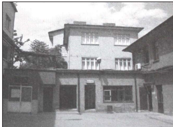
Figure 4.8 Duty House located in the Factory Campus (Source: Cengizkan, 2009, 70)
