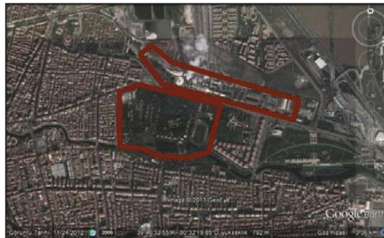
Figure 4.24 Ariel Photography of Factory Campus (Source: Revised by the author)
