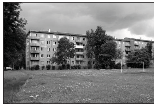
Figure 3.23 Photography of Khrushchevki (Source: http://khrushchevki.wordpress.com/ , accessed in 6 th February, 2013)
