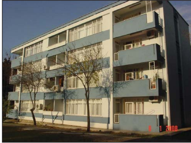
Figure 5.77 Photography of SD block (Source: İSDEMİR Archive, 2012)
