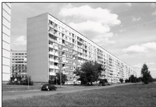
Figure 3.22 Photography of Khrushchevki (Source: http://khrushchevki.wordpress.com/ , accessed in 6 th February, 2013)
