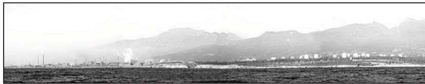
Figure 5.17 Photograph of Factory site from the sea (Source: İSDEMİR Archive, 2012)
