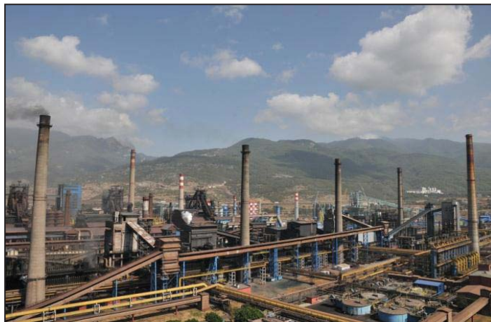
Figure 5.23 Photography of Factory area (Source: İSDEMİR archive, 2012)
