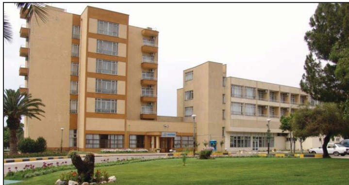
Figure 5.94 Photography of Guesthouse (Source: İSDEMİR Archive, 2012)
