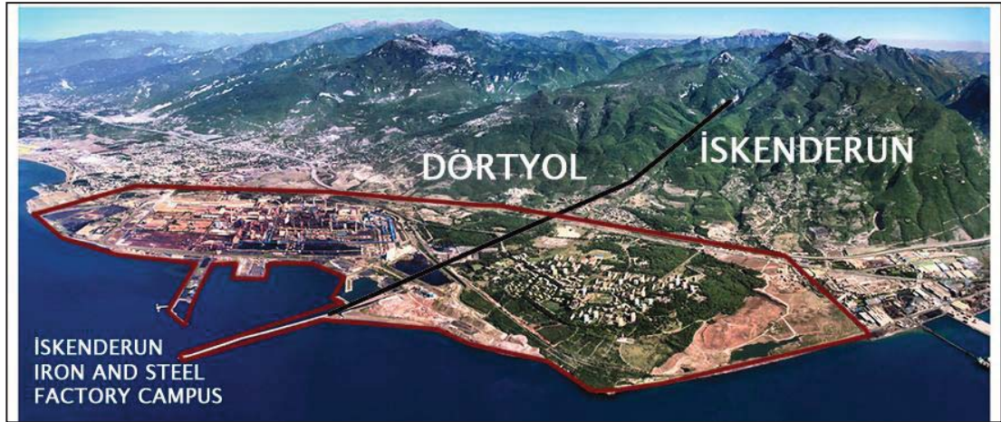
Figure 5.15 Ariel Photography showing borderline of factory campus and administrative bodies
