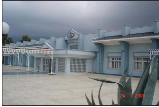
Figure 5.92 Photography of Cultural center (Source: İSDEMİR Archive, 2012)
