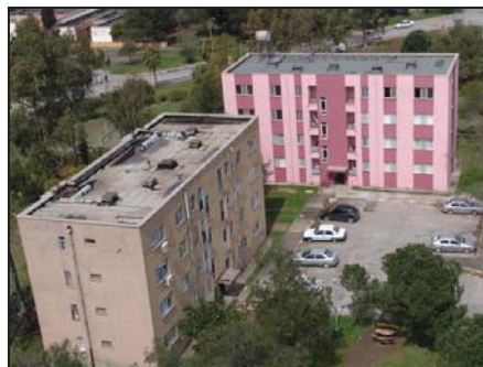
Figure 5.37 Photography of A block (Source: İSDEMİR Archive, 2012)
