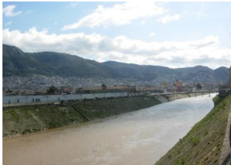
Figure 5.70 A Treeless Riverside – Antakya City Center (Personal Archive, 2010)
