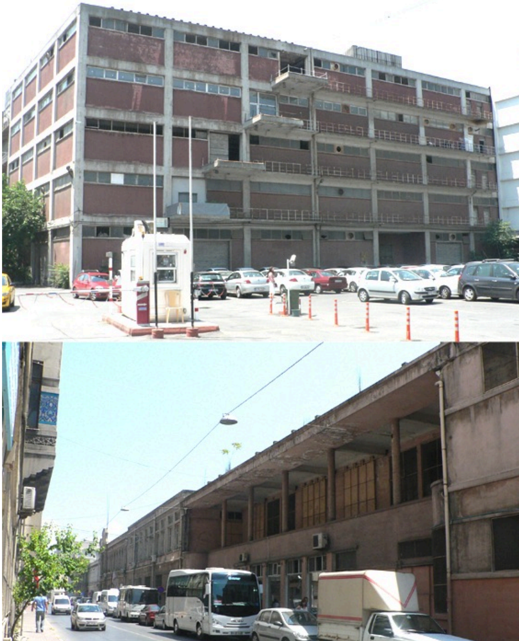
Figure 5.6: Worn out warehouses and historic buildings that need restoration actions.
