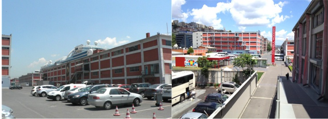
Figure 5.5: The space between buildings is used as parking lots and social activities lacks.
