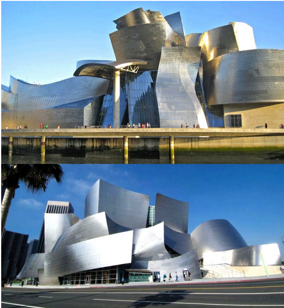
Figure 4.4: Bilbao Guggenheim museum (above) and Los Angeles Walt Disney concert hall. 159 Aren't they similar?
