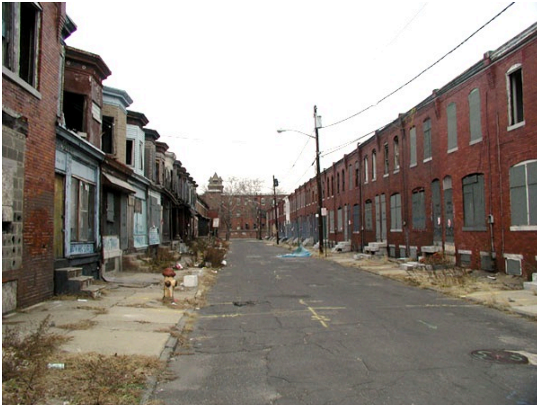
Figure 2.1: Abandoned urban area, Camden, New Jersey. 38
