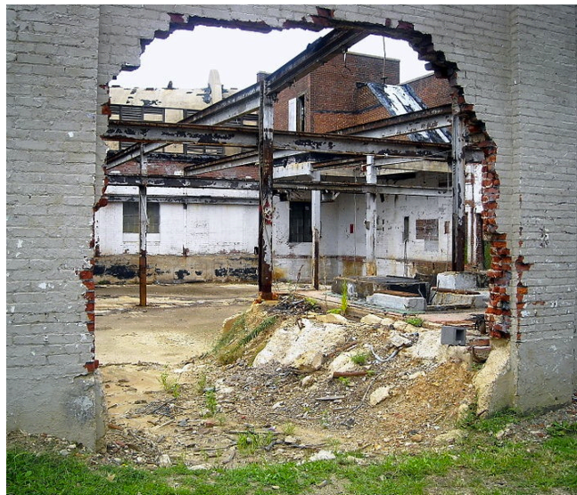
Figure 2.3: An abandoned industrial plant. NoMa, Washington, D.C. 49
