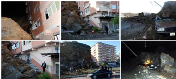
Figure A.5: Zonguldak-Ereğli rock fall on April 21, 2011. The 7-story building and the cars parking around the building were damaged severely, as well as the road was closed due to falling rocks. Source: http://www.dha.com.tr/dhaalbumdetay.asp?kat=12353&page_number=1 (Accessed on April 2011).
