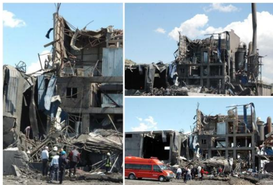
Figure A.8: Industrial explosion in Kahramanmaraş on April 13, 2012. A jean-painting factory exploded and almost 2/3 of the building collapsed killing 4 workers. Source: www.hurriyet.com.tr ; http://www.ntvmsnbc.com ; http://www.stargazete.com (Accessed on April 2012).
