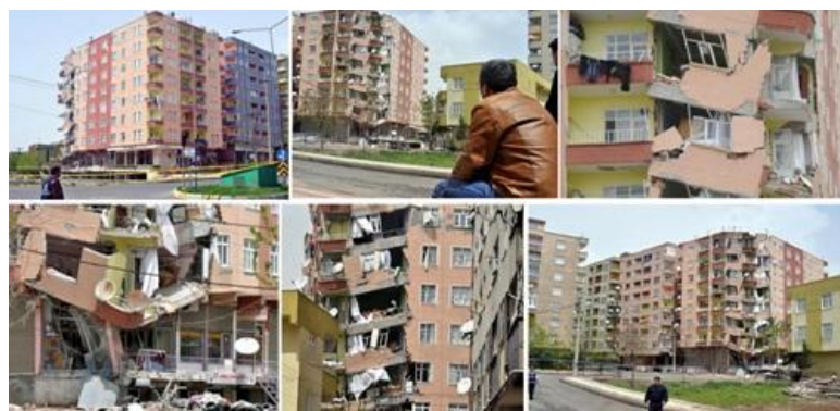
Figure A.6: Boiler explosion in Diyarbakır on April 20, 2011. Source: http://www.dha.com.tr/dhaalbumdetay.asp?kat=12338&page_number=1 (Accessed on April 2011).
