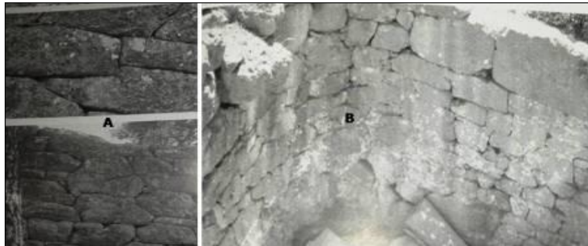
Figure 7.1: Detail From the Joints of a Carian Wall (A) and Fortification Walls (B) (Pimouguet- Pedarros. 2005: 636-637)
