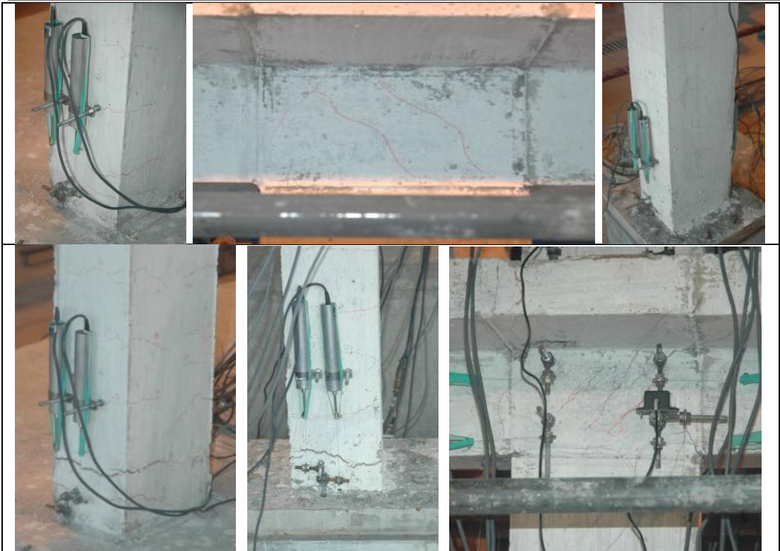
Figure 2. 7 Roof displacement time history/observed damages (SP1)
