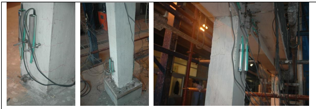
Figure 3. 17 Specimen #1 1 st storey column damages during D2
