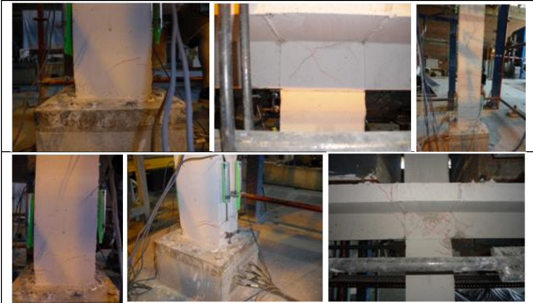
Figure 2. 11 Roof displacement time history/observed damages (SP2)
