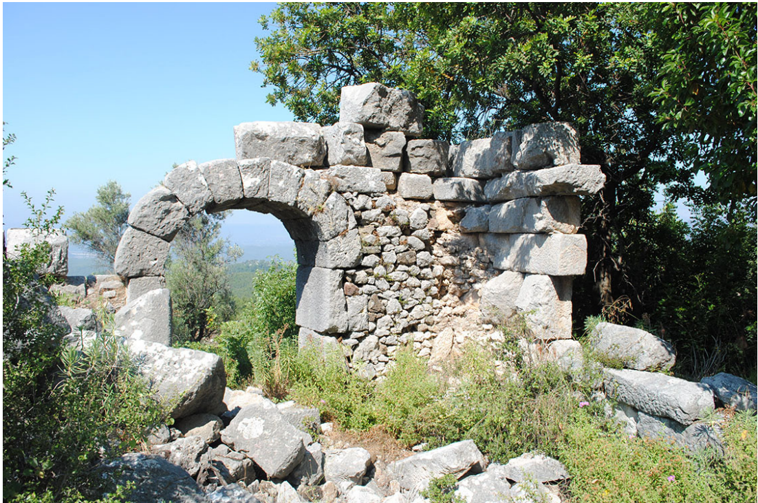
Photo. 34: The bath-house viewed from inside towards southwest. The arched window, rubble inner face and cut stone outer face of the walls are seen.
