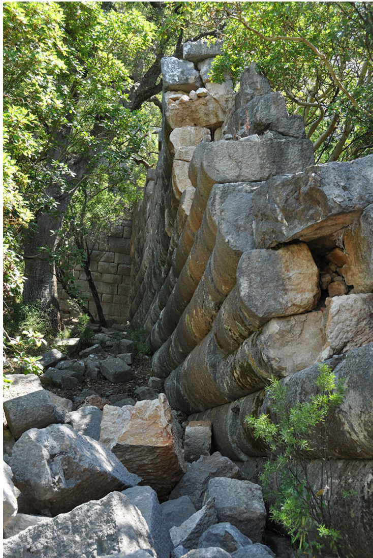
Photo. 23: Pulvinated blocks of the fortifications adjacent to the northern gate. Tower of the northern gate is seen in the background.
