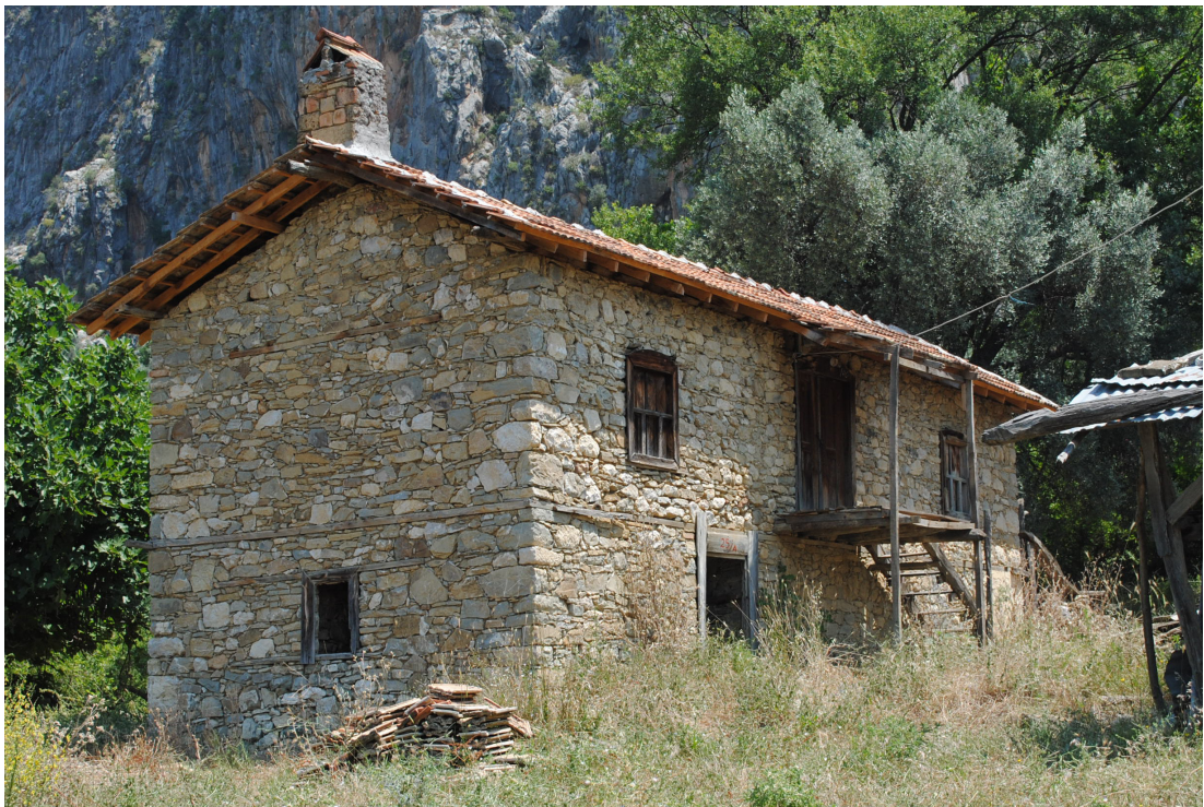
Photo. 63: Another typical example of contemporary vernacular architecture with rubble walls, heavy timber use and pitched roof with ceramic roof tiles.
