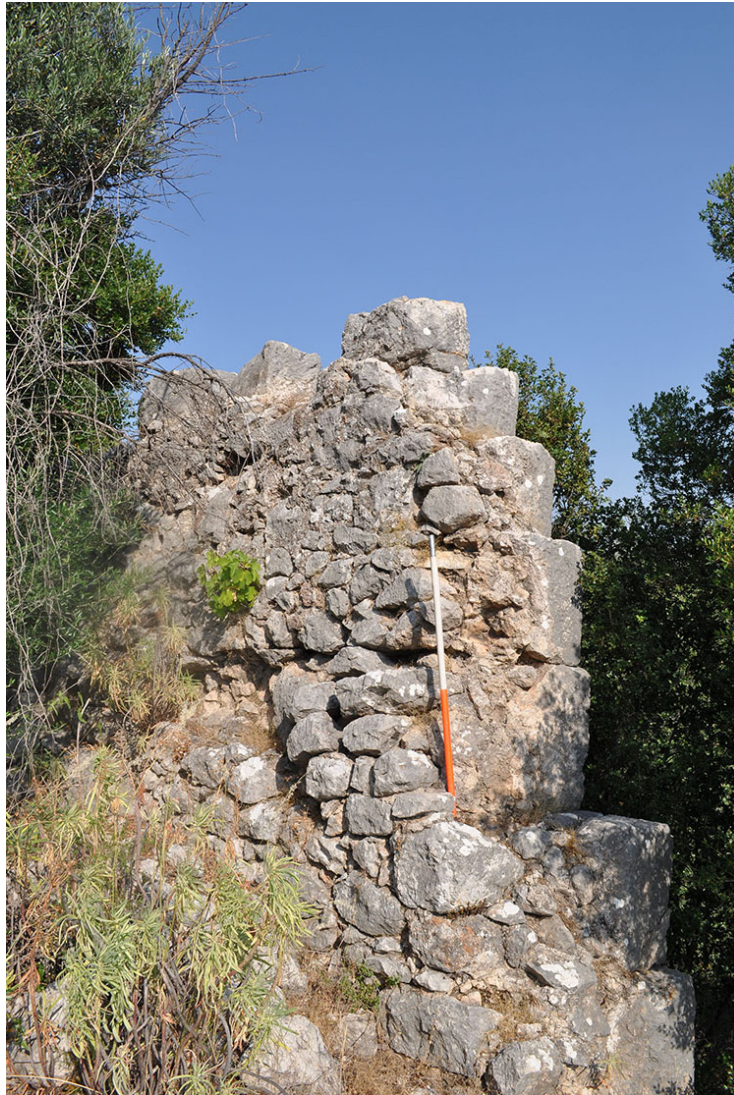
Photo. 42: The temenos wall of the Apollo Sanctuary viewed from inside.
