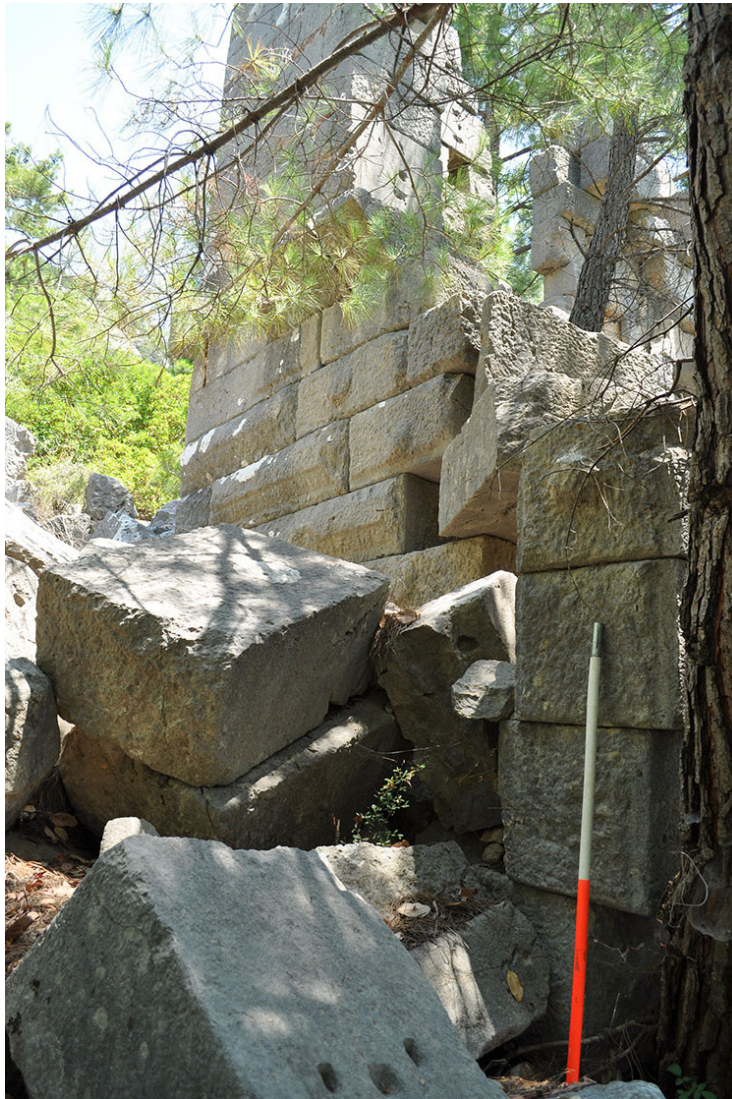
Photo. 10: The western gate and its tower. In the lower right corner of the foreground is the door jamb of the gate, in the background is the tower.
