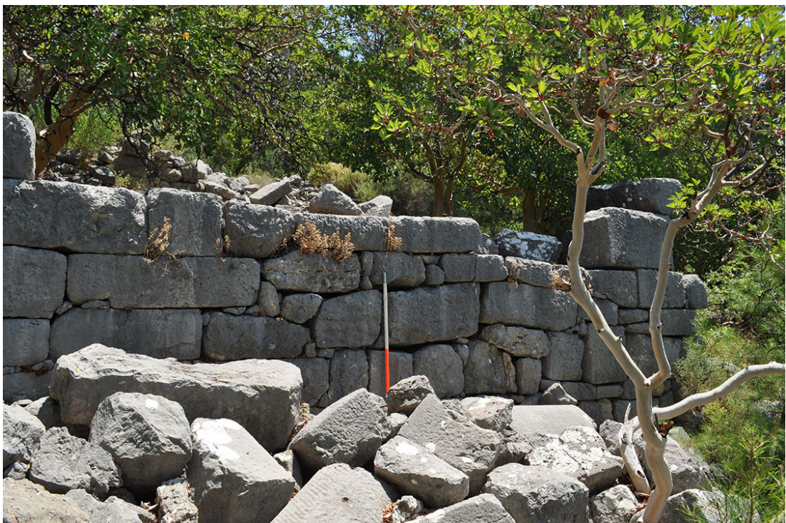
Photo. 21: A later repair/ modification in the fortifications. Compare with photo. 13 and 15.
