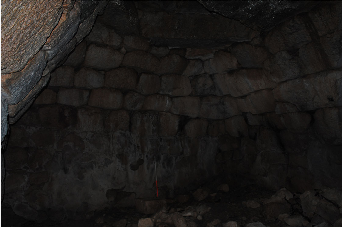
Photo. 48: The chamber in the basement of a house.
