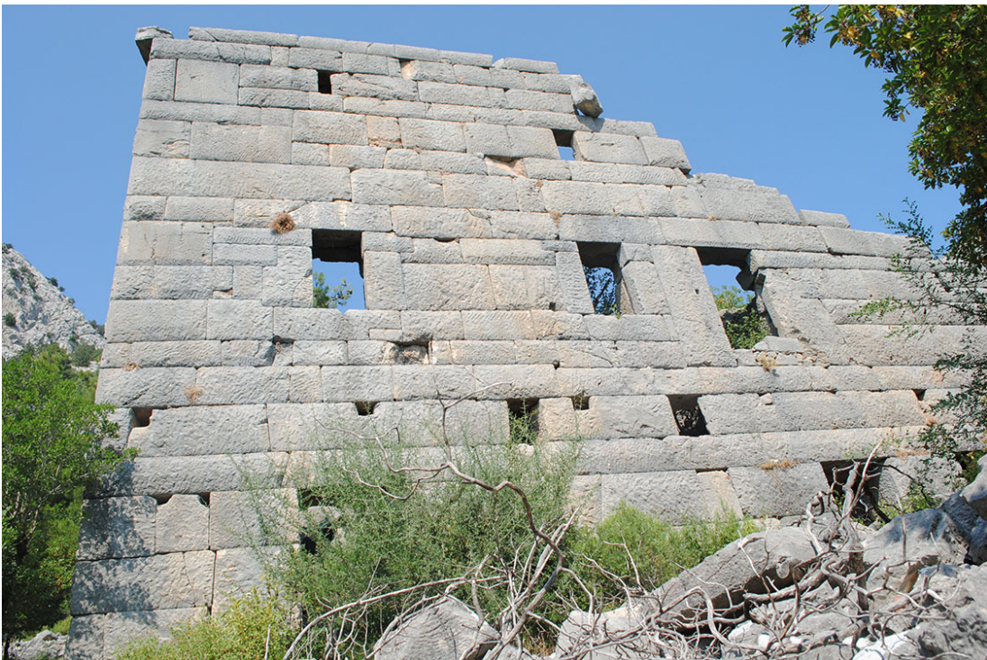
Photo. 29: The southwestern facade of the market building at the northern end of the building.
