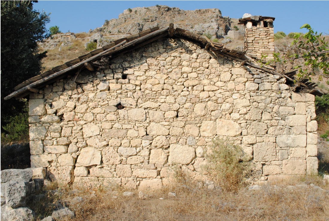
Photo. 68: Another contemporary example with large cut stone blocks in the corners.
