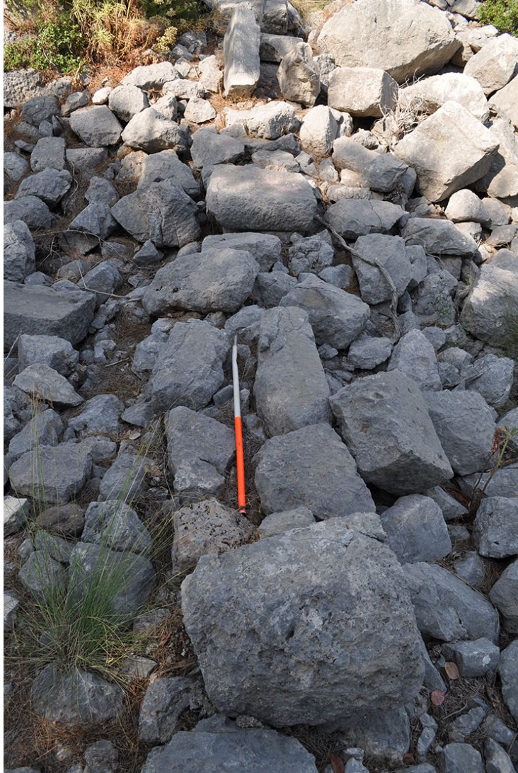
Photo. 55: A typical stretch of an emplekton wall from a domestic context with cut-stone blocks on both faces and earth and rubble fill in between.
