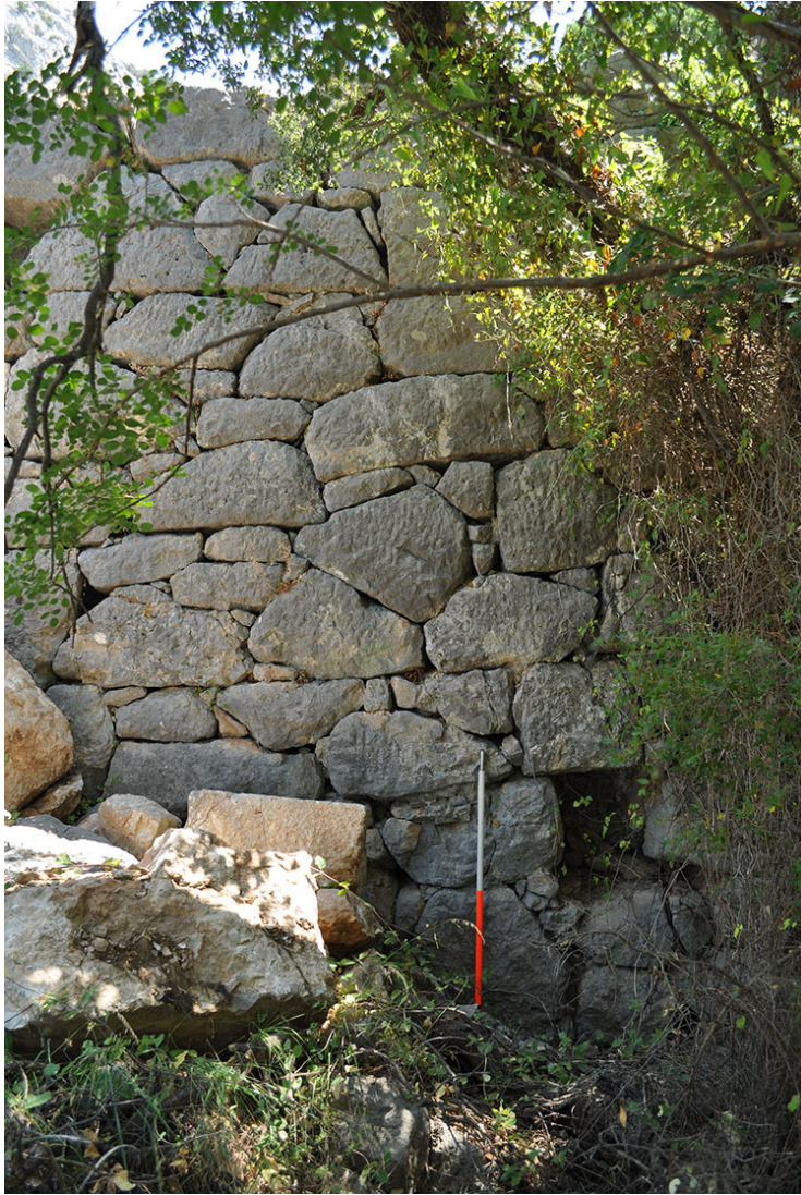
Photo. 31: The terrace wall between the agora and the market building. Compare with photo. 27.
