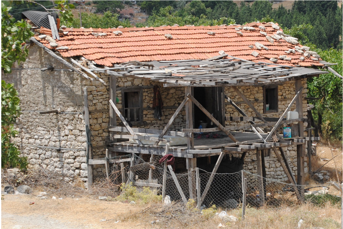
Photo. 62: A typical example of contemporary vernacular architecture with rubble walls, heavy timber use and pitched roof with ceramic roof tiles.
