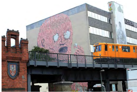
Pin 9. - Pin 10. Oberbaum Bridge/ River Spree
