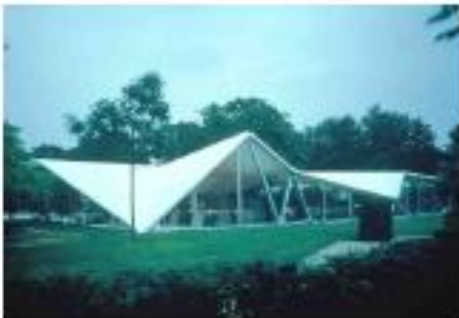
Serpentine Gallery Pavilion 2000 Designed by Zaha Hadid
