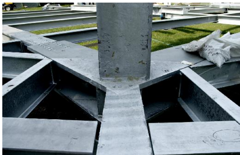
Figure 43 Welded Details of Steel Column.
