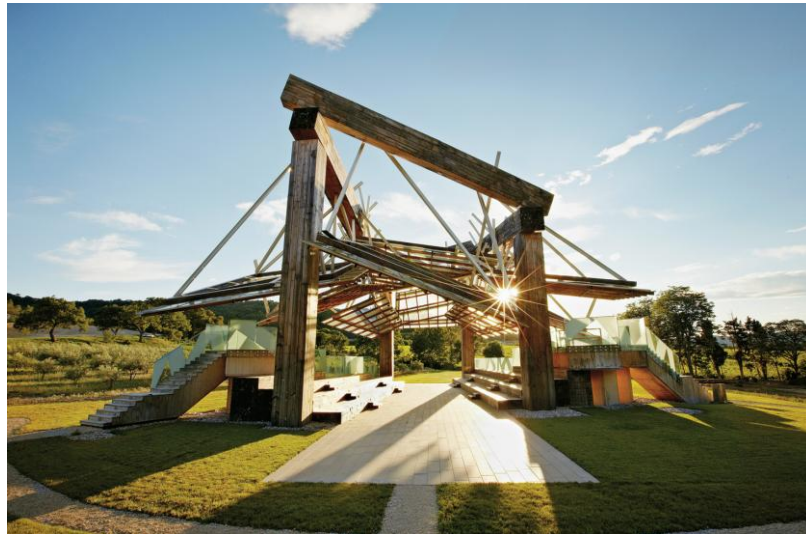
Figure 28 The 2008 Serpentine Gallery, relocated to the Château La Coste winery, Aix-en-Provence, France.
