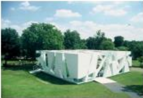
Serpentine Gallery Pavilion 2002 Designed by Toyo Ito with Arup
