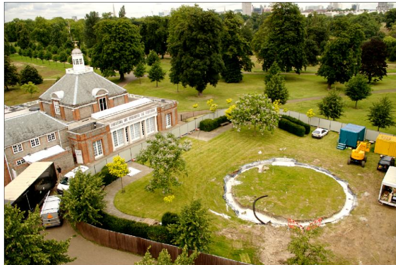
Figure 48 Excavation Site of the 2007 Serpentine Pavilion.
