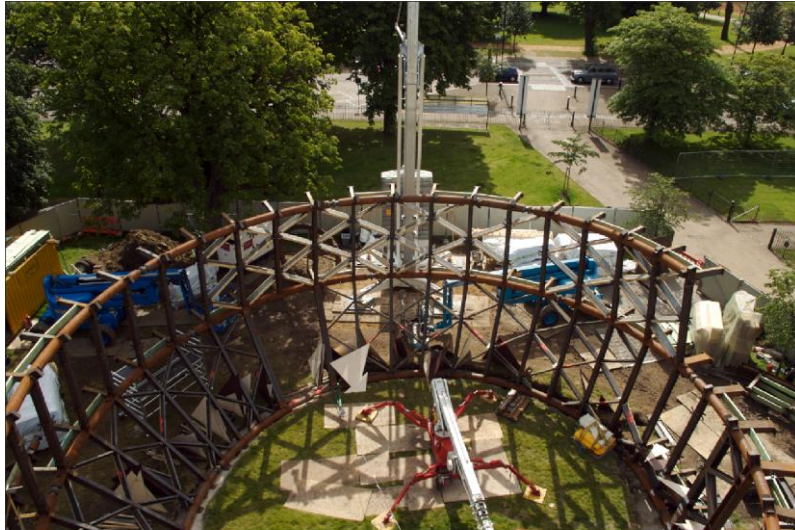
Figure 50 Construction of Circle Steel Structure.
