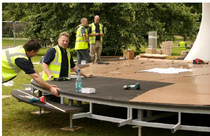
Figure 47 Construction of Wooden Pavement.
