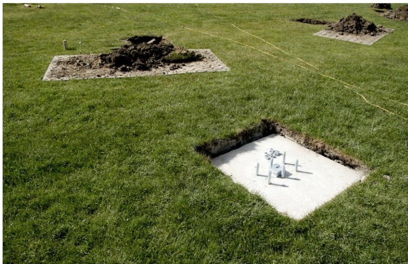
Figure 41 Concrete Footings Detail.
