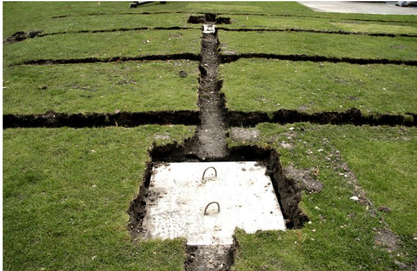
Figure 40 Excavation of Lintel.
