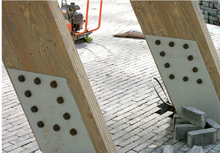
Figure 38 Connection Details between Wood and Steel.
