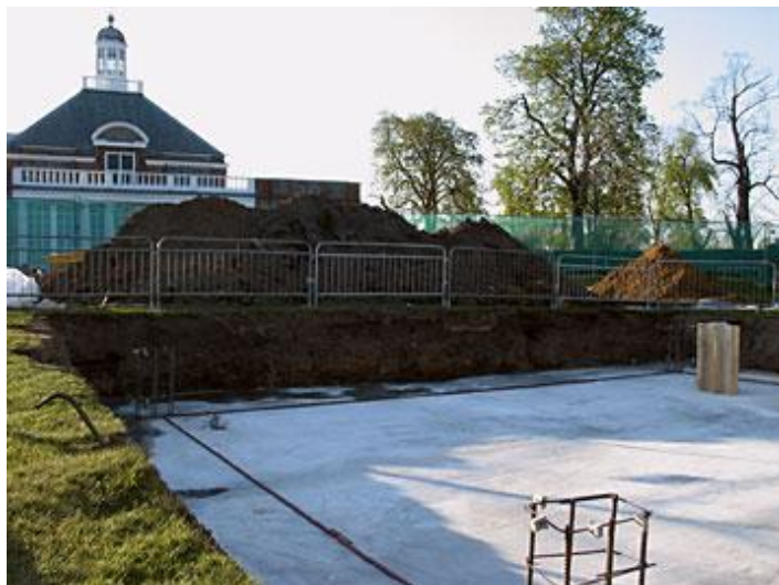
Figure 32 Construction of Concrete Basement.
