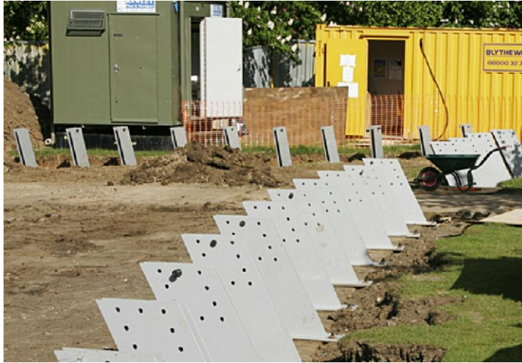
Figure 36 Construction of Steel Connection Elements.
