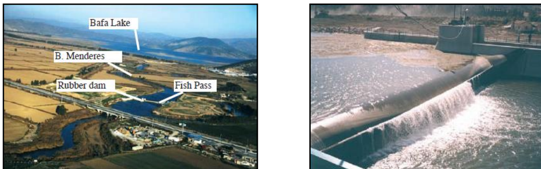
Figure 25. Rubber dam in Bafa Lake
