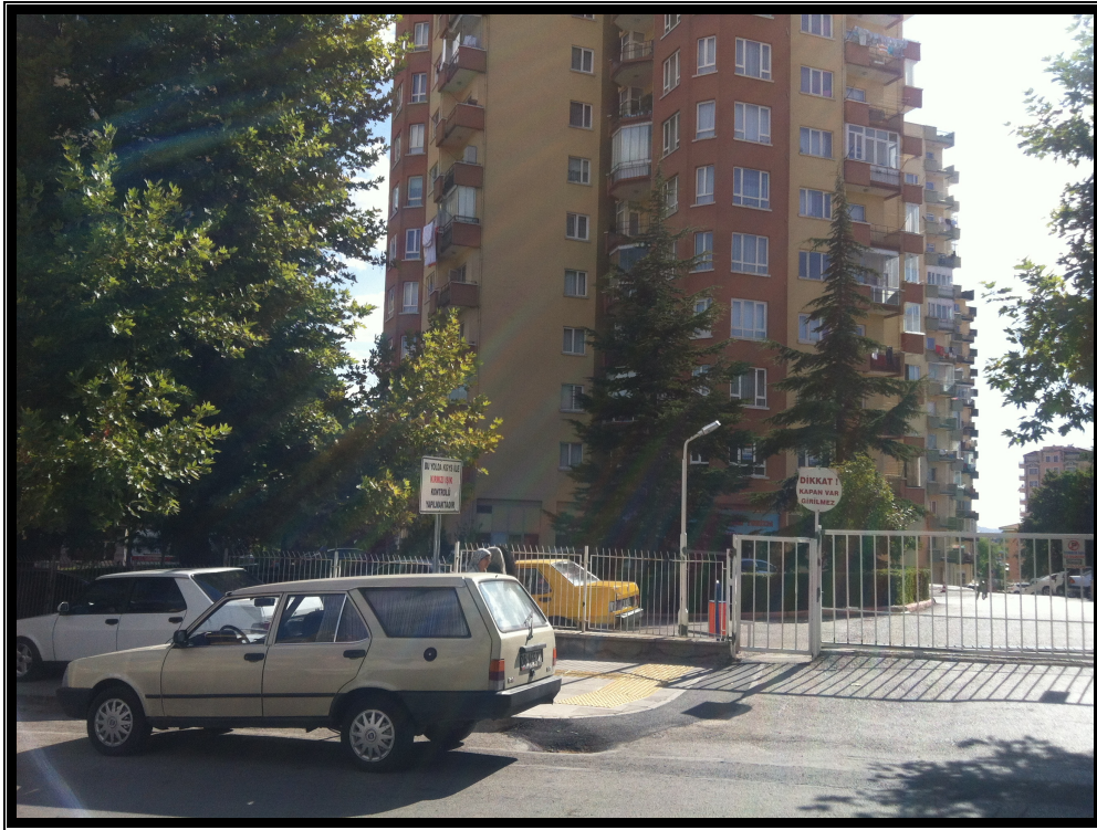
Figure 6.10 A view of Entrance Providing Access Control
