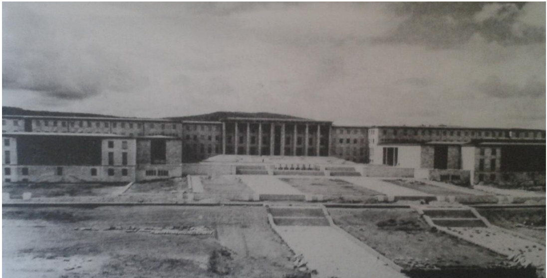
Figure 5.8b: National Assembly Building Construction-2
