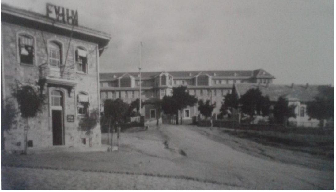
Figure 5.12b: Ankara Numune Hospital (1933)
