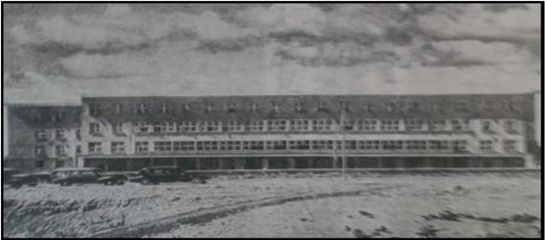
Figure 4.2b: Side View of Maliye Okulu in Ankara (1943-1944)
