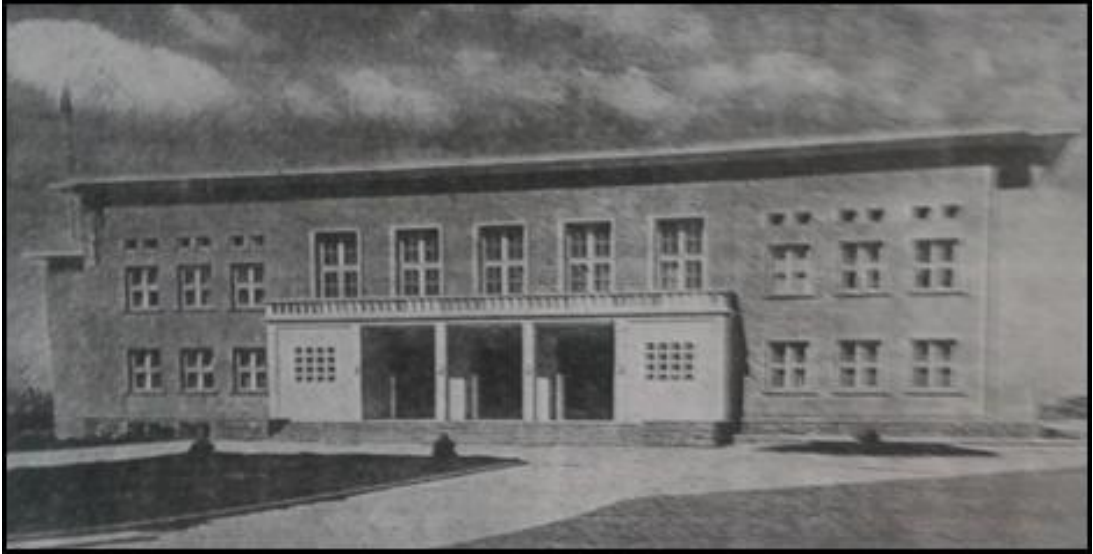
Figure 4.2a: Front View of Maliye Okulu in Ankara (1943-1944)
