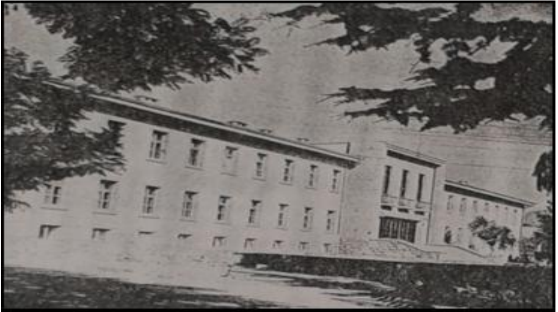
Figure 2.3b: Kayseri Government Mansion Building (1936)
