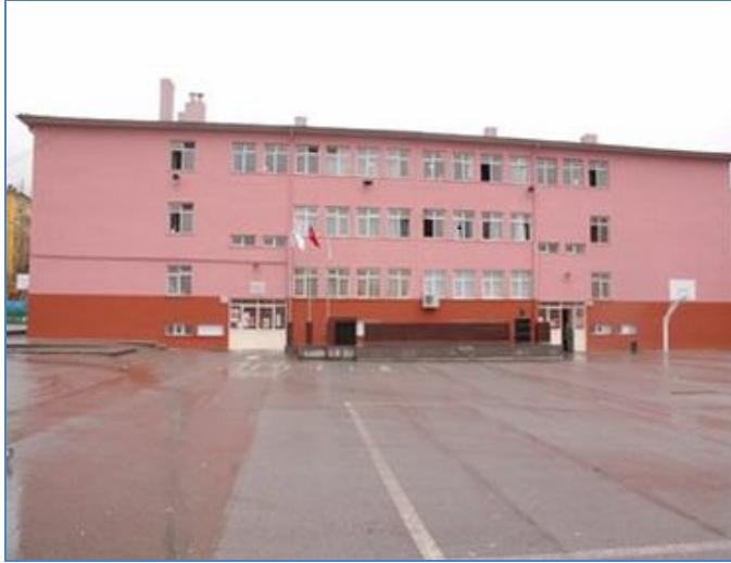
Figure 5.11: Other Group's School Building (Taken by the Author)
