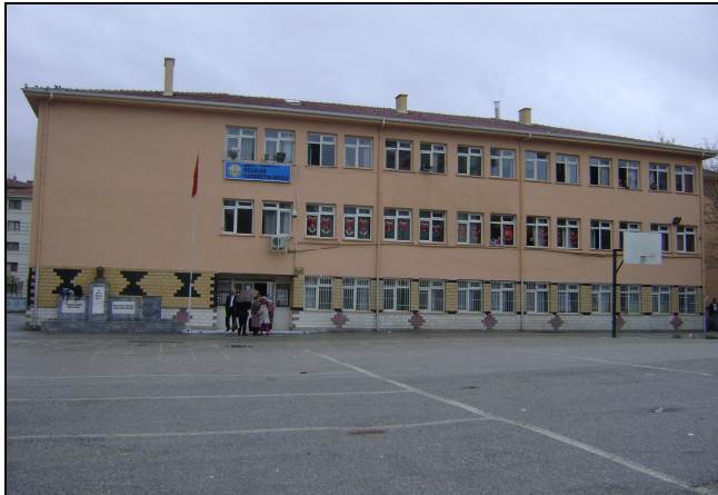
Figure 5.8: Main Group's School Building (Taken by the Author)
