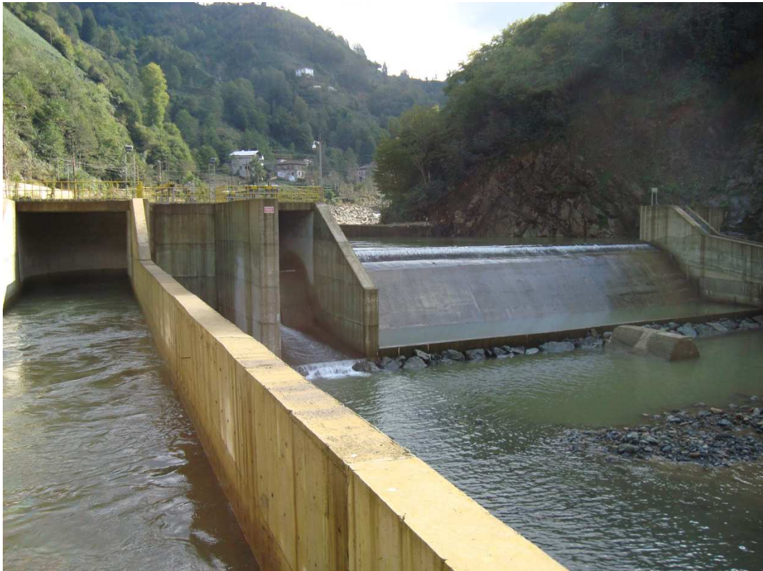
Figure 56 : General layout of Kale Weir and HEPP
