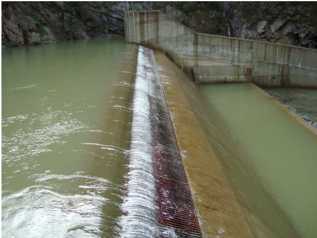
Figure 57 : Trash rack of Kale Weir and HEPP
