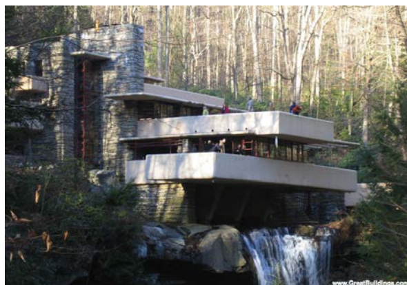
a) Fallingwater (greatbuildings.com)
