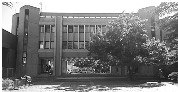
Figure 3.12: The Bridge Building (Site D), which stands above the entrance floor preserving the transition on the alley (an assumption) (Source: Author Photo Archive, 2013)
