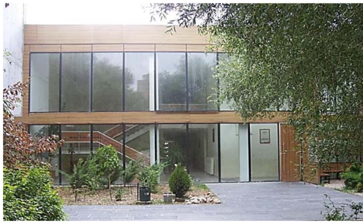
Figure 3.2: Site A_ Department of Basic English: F&G Buildings (Source: Author Photo Archive, 2013)
