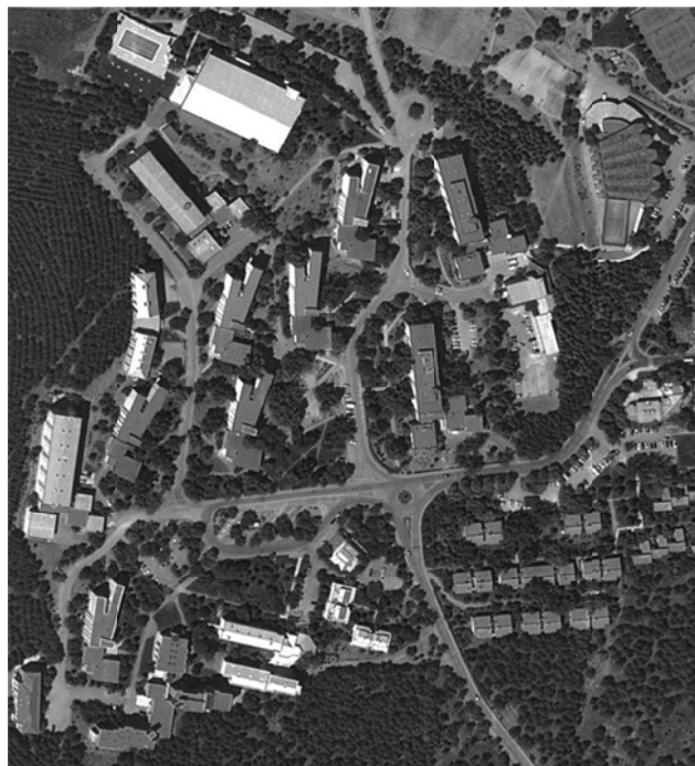
Figure 3.4: Site C_ the Accommodation Zone: Dormitories (Google Earth View, 2013)
