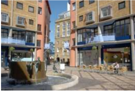
Figure 3.7. Renovation and New Development in Horsleydown Square, Shad Thames, London (Retrieved from; http://www.beenthere-donethat.org.uk/london/london-towerhill059big.html )
