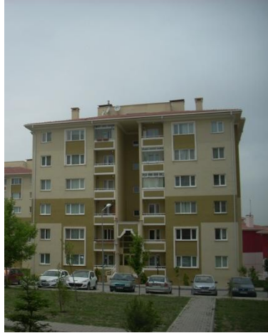
Figure 3.3 Photo of the case study: Building type C, block 10
