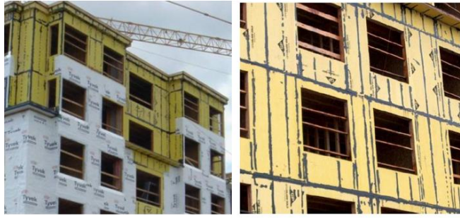
Figure 2.20 An exterior air barrier approach in a Multi-Family Residential Buildings (RHD Building Engineering Ltd., 2013).
