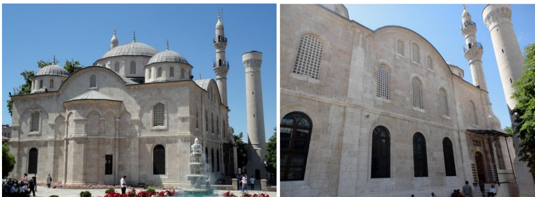
Figure. 169 Left: The south facade of Malatya Yeni Mosque. Right: The east facade of Malatya Yeni Mosque. Author 2011.
