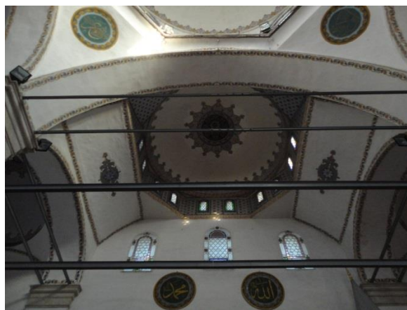
Figure. 124. The dome and the transition element of the cover of Balıkesir Zağnos Pasha Mosque's mihrab section. Author 2011.
