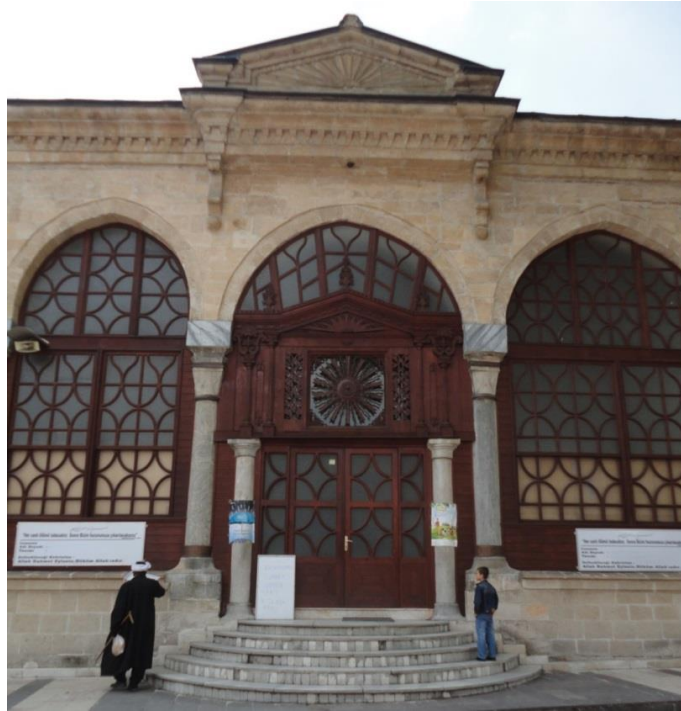
Figure. 53 The triangular pediment on the north facade of the Kütahya Great Mosque. (Author 2011)
