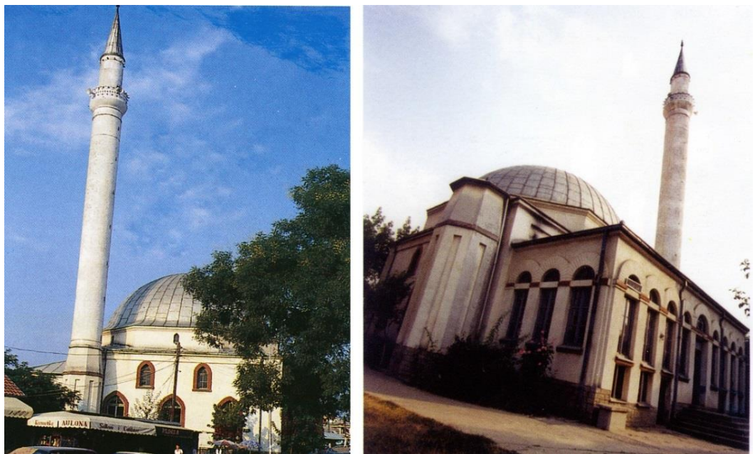
Figure. 175 Left: The west facade of the Firzovik Great Mosque. Right: The north facade of the Firzovik Great Mosque. Source: (İbrahimgil and Konuk 2006, 199)
