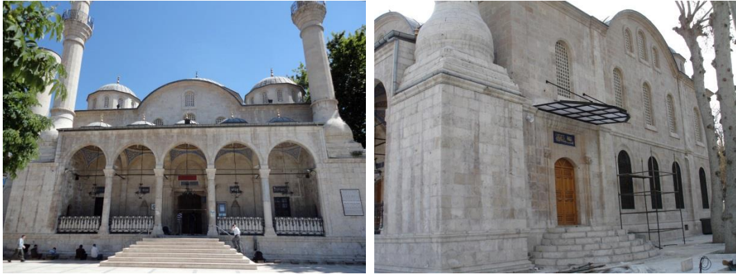
Figure. 170 The north facade of Malatya Yeni Mosque. Right: The west facade of Malatya Yeni Mosque. Author 2011.
