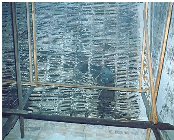
Figure. 127 The half barrel vault on the north side of the Zağnos Pasha Mosque during the restoration work in the 1980's. The brick and the timber frame can be seen. Source: VGM Archive, retrieved in 2011.
