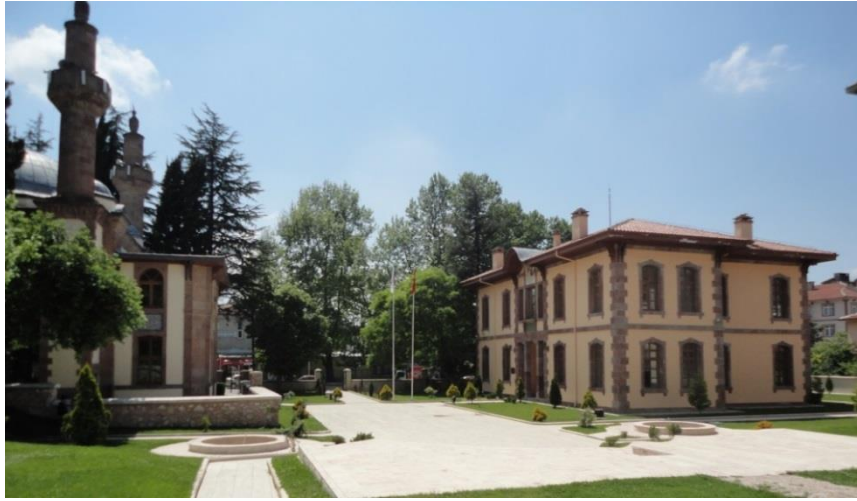
Figure. 155 Sögüt Hamidiye Mosque on the left and Sögüt Hamidiye High School on the right. Author, 2011.
