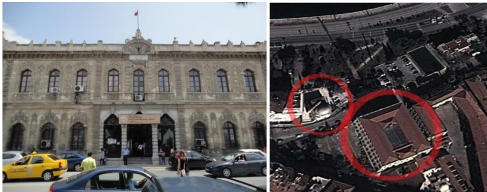
Figure. 61 Left: İzmir Mithat Pasha Sanayi Mektebi (Occupational Art and Craft School), (Author 2011), Right: Hamidiye Mosque on the left hand side and Art and Craft School on the right hand side, retrieved from www. maps.google.com , in June 2013.
