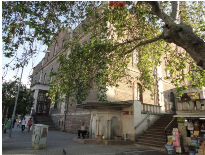
Figure. 126. Balıkesir Zağnos Pasha Mosque from north-east corner. Author 2011.
