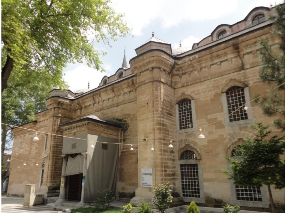
Figure. 51 The west entrance and facade of the Kütahya Great Mosque. (Author 2011)
