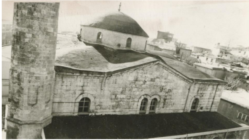
Figure. 78 The north facade of Adiyaman Great Mosque, 1983. Source: VGM Archive, retrieved in 2011
