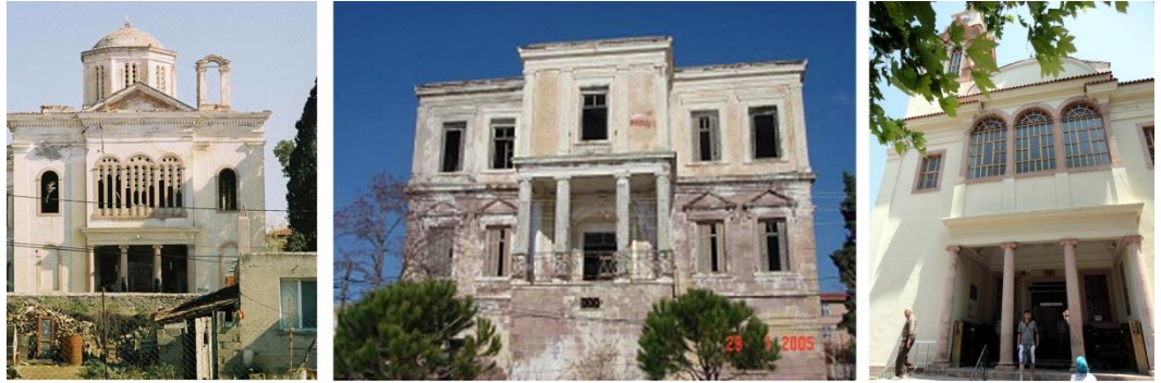
Figure. 97. Images from left; Taksiyarkis Church in Cunda, Despot's Villa in Cunda and Hagia Ioannes Church (Saatli Mosque) in Ayvalik. Sources respectively; Erdem, Özakin, Yergün, 2007, p. 93, 94 and author 2011.
