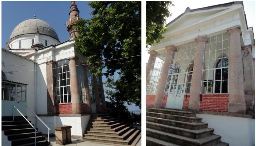
Figure. 91 The elevated last prayer hall of the Ayvalık Hamidiye Mosque (Author 2011)
