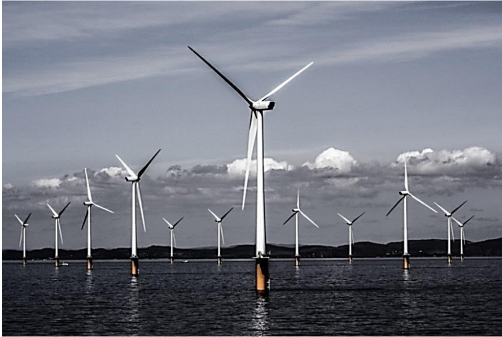
Figure 1.12 Modern Offshore Wind Turbine [32]
