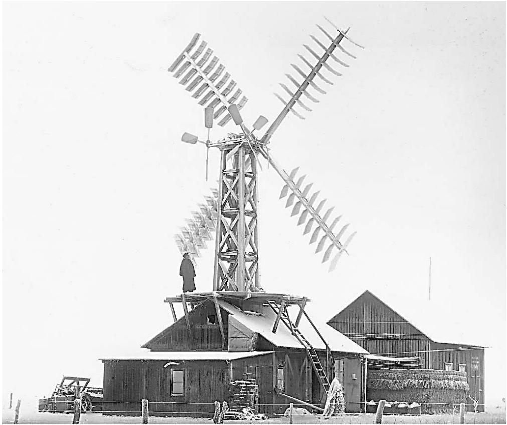
Figure 1.11 La Cour's First Electricity Producing Wind Turbine in 1891, Askov, Denmark [1]
