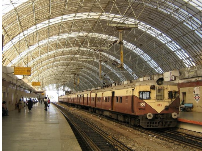
Figure 5-11: The platform shelter at Thirumailai Station, LUZ, Chennai, India
