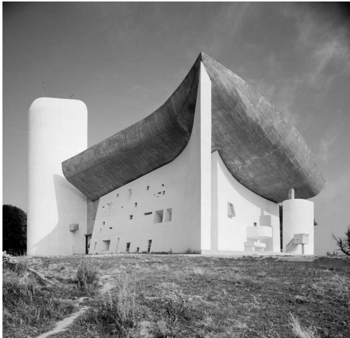
Figure 3 Le Corbusier, Chapel of Notre Dame Du Haut, 1955, Ronchamp. From: http://www.1stdibs.com/art/photography/black-white-photography/ezra-stoller-notre-dame-du-haut-ronchamp-chapel-le-corbusier-ronchamp-france/id-a_43664/ , accessed October 06, 2013.
