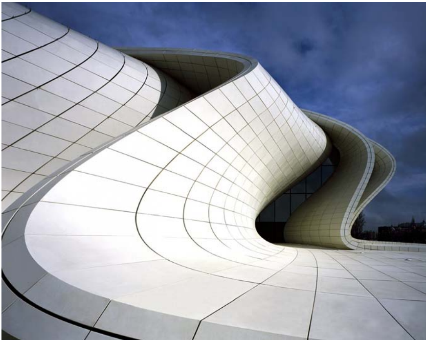
Figure 20 Zaha Hadid, Heydar Aliyev Cultural Center, folds of the envelope. From: http://www.zaha-hadid.com/architecture/heydar-aliyev-centre/ , accessed September 09, 2013.
