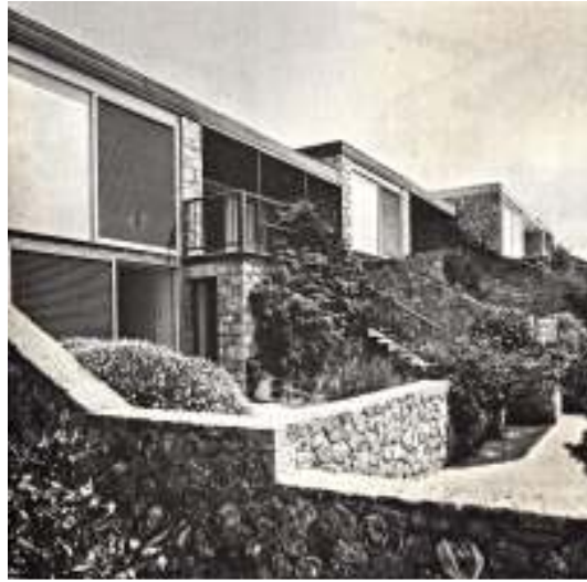
Figure 3 15 A house in Apollonion by Doxiadis Associates in Porto Rafti, Greece (1975).
