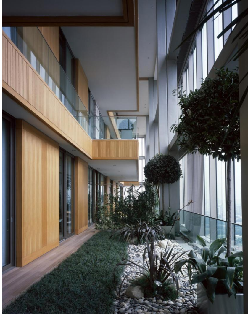
Figure B.4 A view from the east facade (Source: Tabanlıoğlu Architects)
