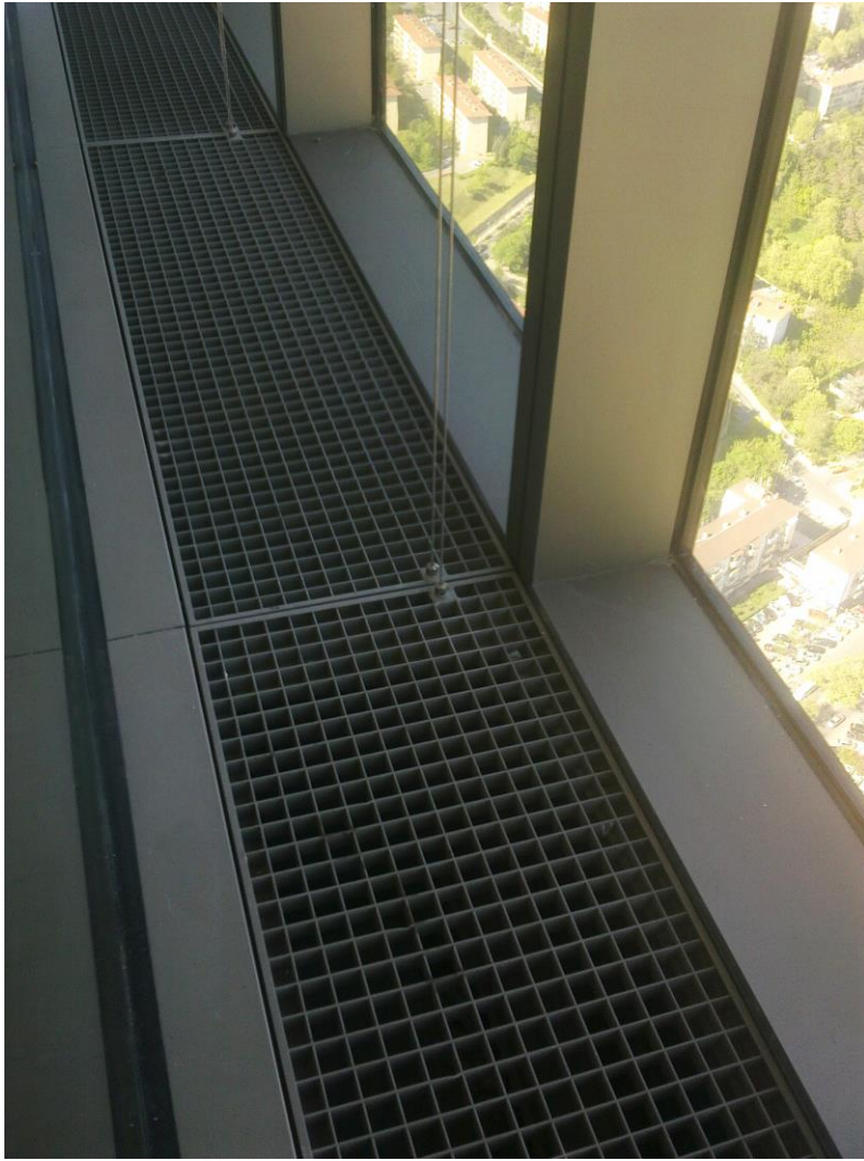
Figure B.8 A view of the inlets
