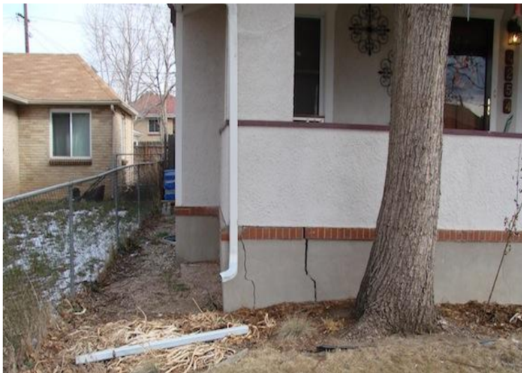
Figure 1.3. A View of Damage of a Building due to Expansive Soil (source: http://www.montrealhomeinspectorpro.ca/en/home-inspection-articles/view/560/Visual-Inspection-of-Concrete )
