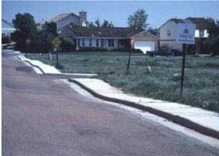
Figure 1.2. A View of Road Undergoing Swelling (source: http://geosurvey.state.co.us/hazards/Swelling%20Soils/Pages/Definition.aspx )
