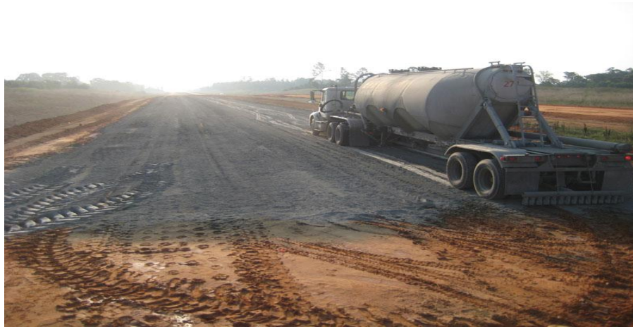
Figure 2.14. A View of Stabilizing Expansive Soil with Cement (source: http://www.ctre.iastate.edu/research/detail.cfm?projectID=-373342403 )
