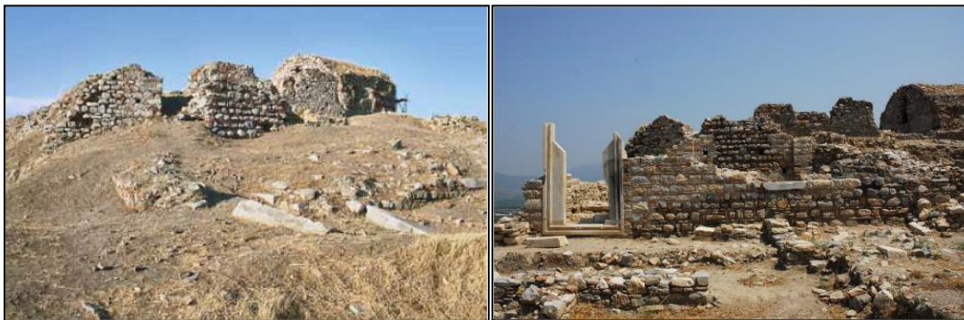
Figure 3-34: The ‘Köşk’ before and after the restoration work (Source: Büyükkolancı,2009)
