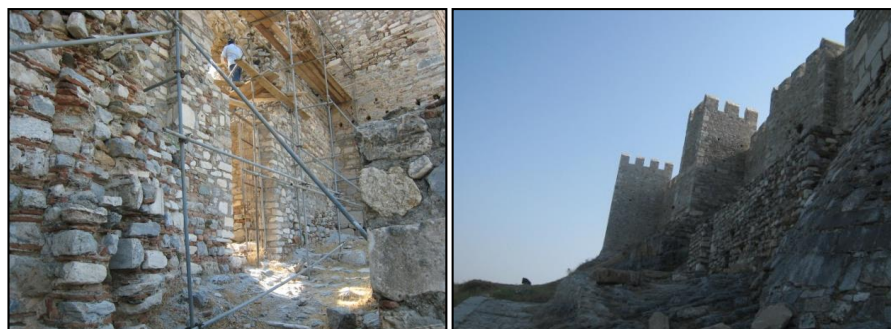
Figure 5-18 Restoration on the western Fortress Walls (Personal archive)
