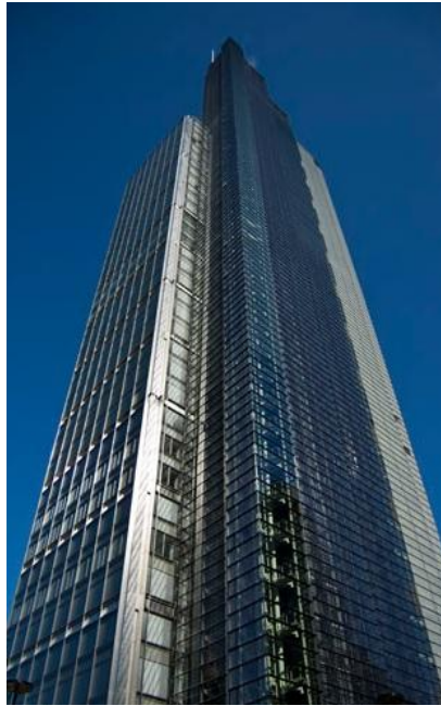
Figure 2.40. The Heron Tower, London (Source: http://photography.jfranklin.com )
