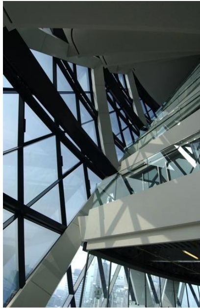
Figure 4.30. Triangular form of the windows (Source: www.fosterandpartners.com )
