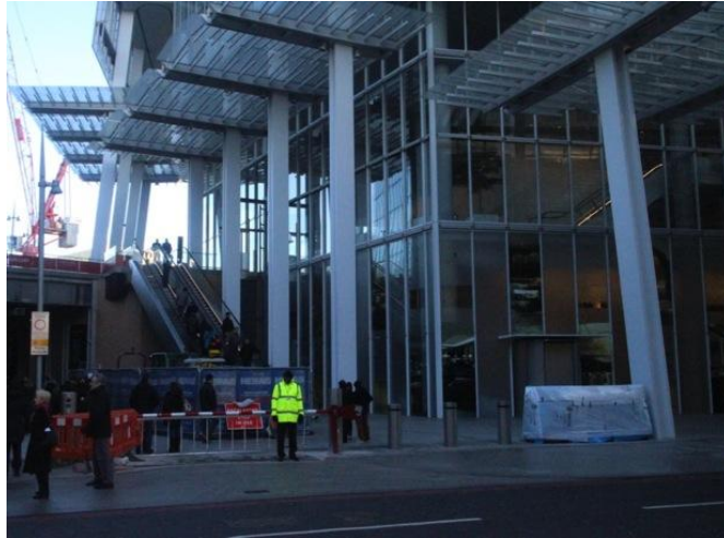
Figure 4.10. Façade material usage on the entrance floors of The Shard: transparent and frosted glass. (Archived by Author)
