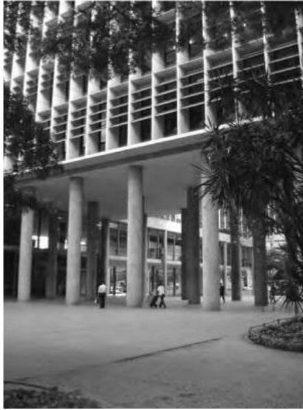
Figure 2.43. The ground floor of Ministry of Culture and Education in Rio de Janeiro and the open public space created by the podium and the pilotis 1 through which pedestrians can cross the urban block (Source: Gonçalves, 2010)
