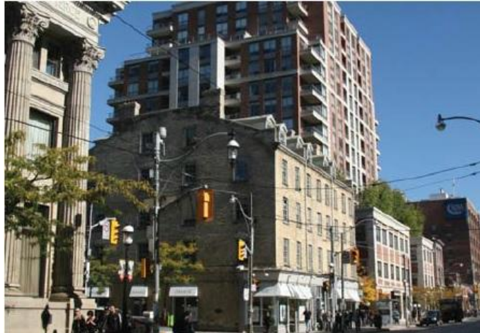
Figure 2.28. The historic streetwall context is respected with a generous tower stepback and referenced through an appropriately scaled and articulated base building (Source: Tall Building Design Guidelines, 2013)
