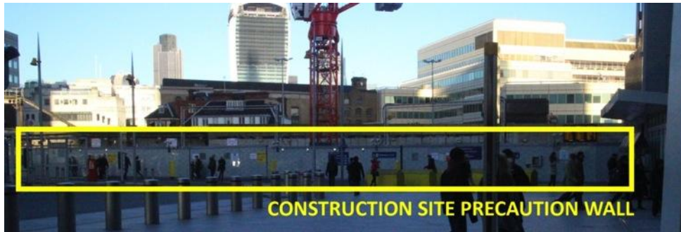
Figure 4.18. Construction site and precautions (Archived and Drawn by Author)
