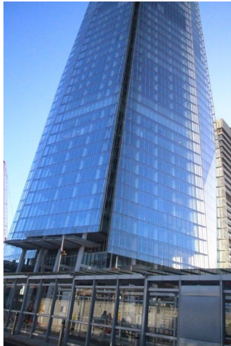
Figure 4.9. Picture showing The Shard’s façade material usage; extra white glass (Archived by Author)
