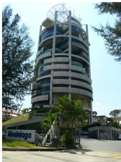
Figure 2.45. Menara Mesiniaga, a bioclimatic building in Kuala Lumpur (Source: www.solaripedia.com )
