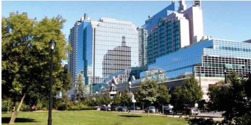
Figure 2.20. Tall buildings designed to protect sunlight and sky view in a public park (Source: Tall Building Design Guidelines, 2013)
