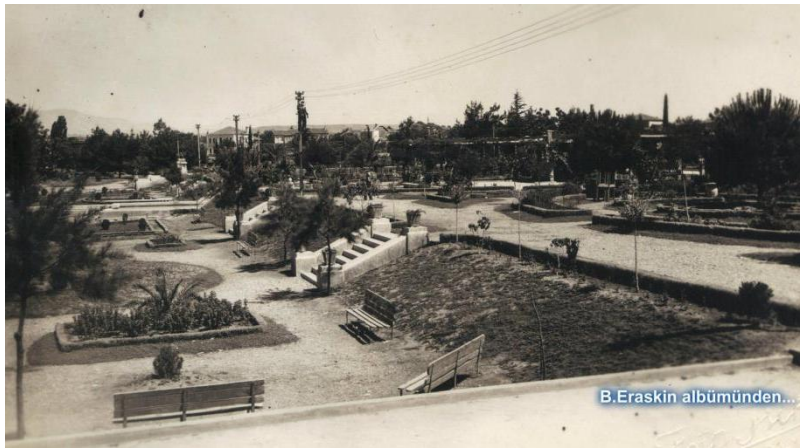
Figure 3.2. Karaaliođlu Park in the 1940s (Source: personal archive of B. Eraskın)
