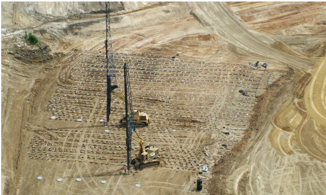
Figure 2.5. Mandrel-installed wick drains at a site
