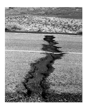
Figure 2.3 An example of a severely developed thermal crack in an asphalt concrete pavement.
