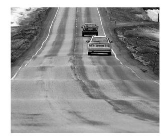
Figure 2.4 The effect of frost action on asphalt concrete pavements.
