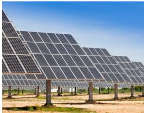
Figure 2.1.b. Solar panel configuration with solar tracker system (Heliostats)
