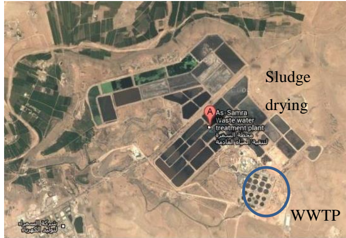
Figure 4.12 As-Semra WWTP in Jordan (Google map)
