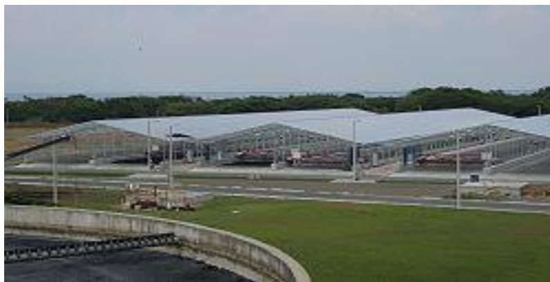
Figure 2.11 Another view of the solar sludge drying plant in Managua/Nicaragua (Scharenberg et al., 2010)
