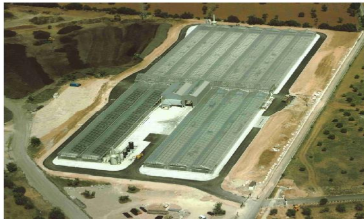
Figure 2.9 A view of Palma de Mallorca greenhouse solar drying plant in Spain with 20 000 m 2 area, (Ritterbusch et al., 2012)
