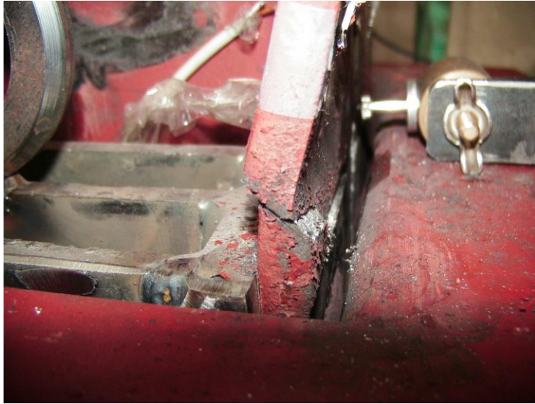
Figure 7.5. Side view of fracture occurs above the 400 mm-high steel base fixture.
