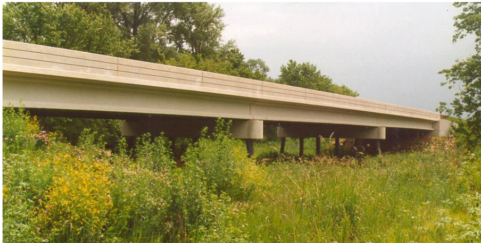
Figure 2.4. Bridge #55555 in Olmsted County, Minnesota over the Zumbro River
