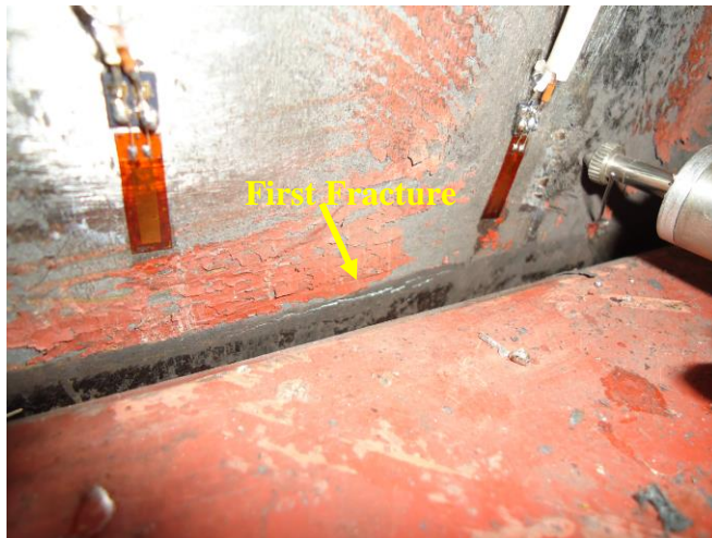
Figure 7.9. First fracture occurs 220 cycles.
