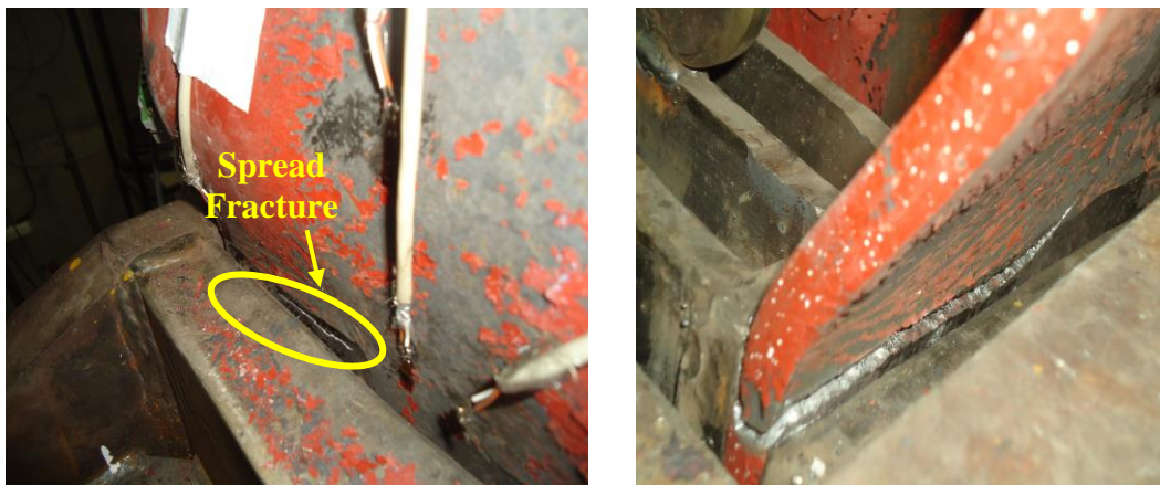
Figure 7.62. Spread fracture and close view of the crack.
