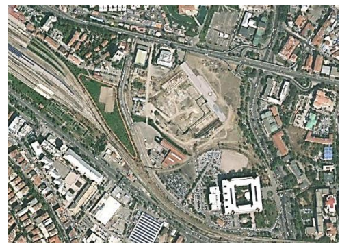
Figure 44 - How the site looked like until 2011, as a void (Google Earth Image, 17/09/2010)
