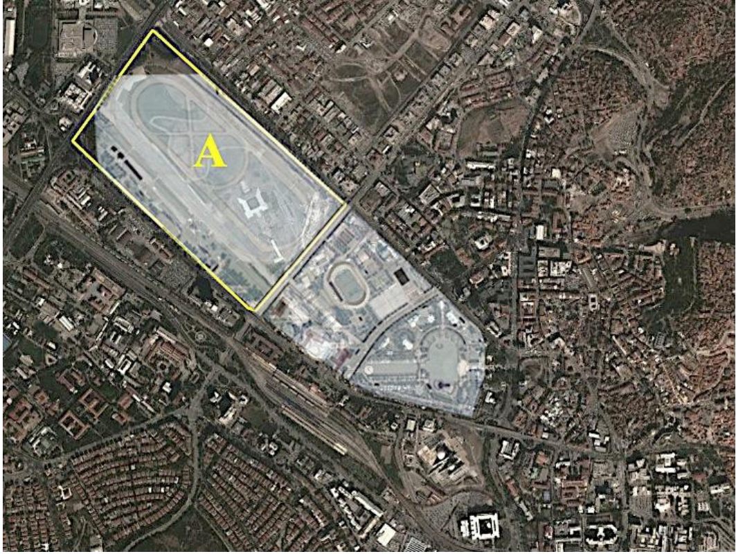
Figure 66 - Yücel-Uybadın plan superimposed on the current aerial view of the site (Processed with Figures 45 & 65)
