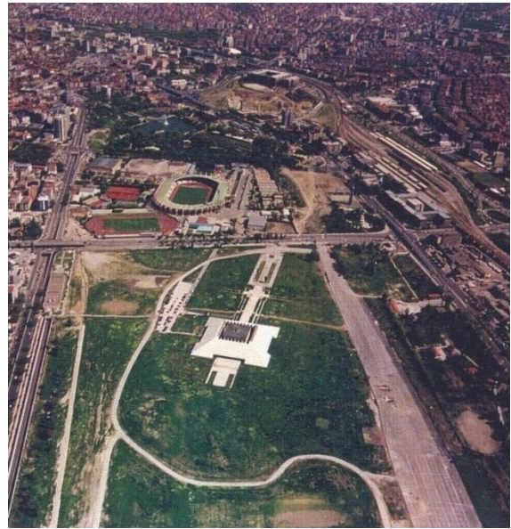
Figure 88 - AKM Building and Areas Aerial View (Filiz & Coşkun Erkal archive)
