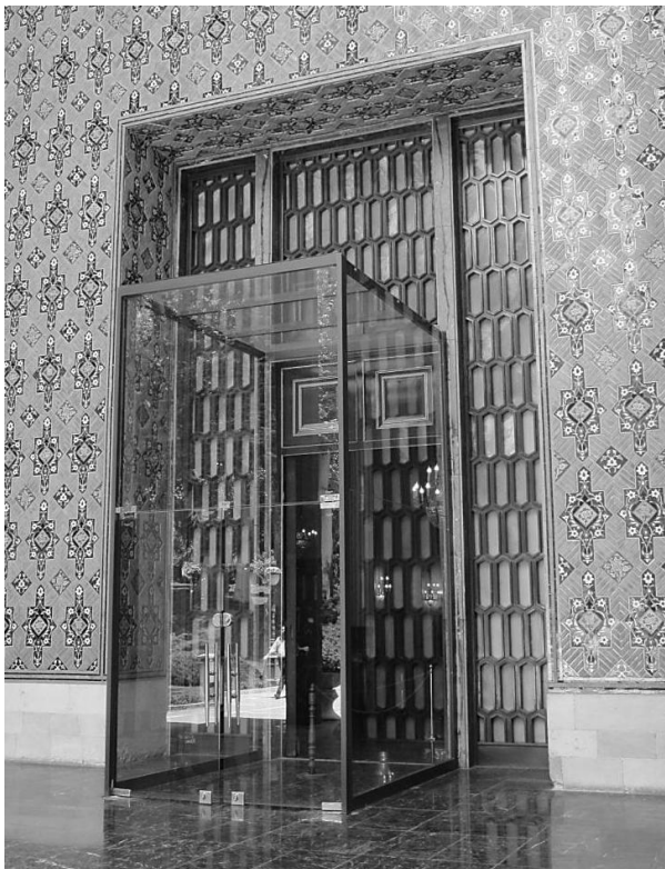
Figure 205 A detailed view from the main entrance of the Palace of Niavaran, 2011.
