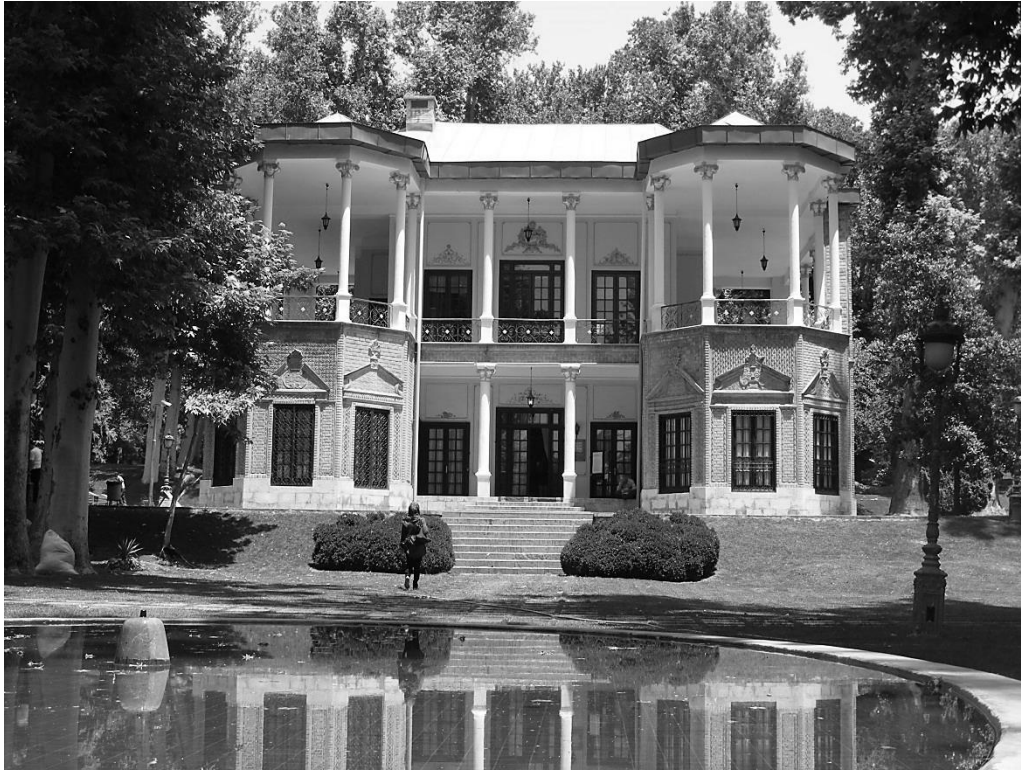
Figure 201 View of the Ahmad-Shahi Kiosk, the Niavaran Palace Complex, 2010. SOURCE: Author, 2010.
