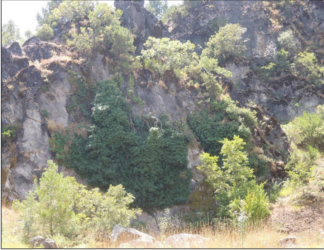
Figure 3-8: General view of steeply sloping fault scarp of the Küçüktaštepe fault (near north of Küçüktaštepe Hill, view to southwest)
