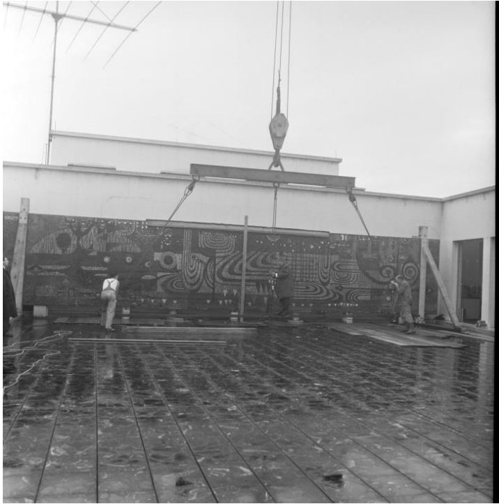
Figure 212. Dismantling the mosaic. Source: NATO archives
