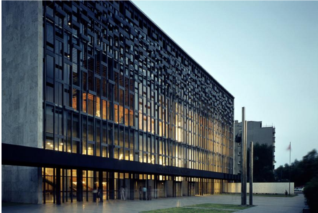
Figure 161. The entrance area of AKM Building Source: SALT Reseach Archive
