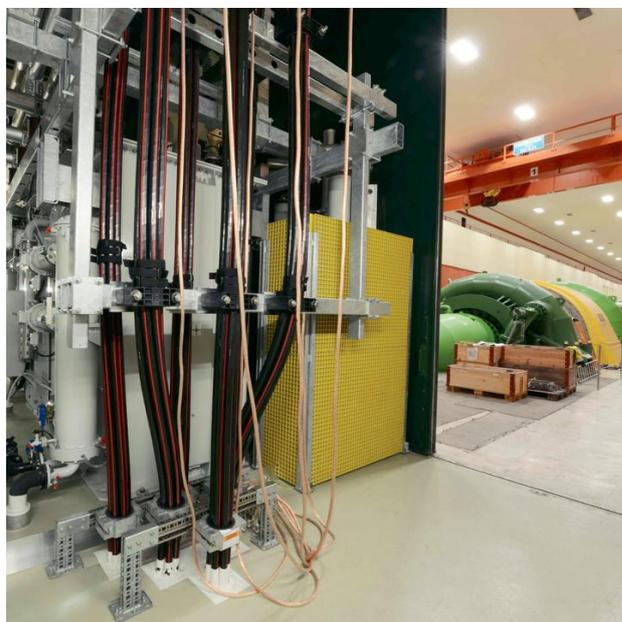
Figure 1.6 MMC based motor drive for a converter-fed synchronous machine by ABB and Oberhasli Hydroelectric Power Company in Switzerland [11]
