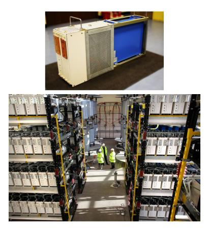
Figure 1.5 Submodule (up) and MMC (down) structure of MaxSine (Alstom) [7]
