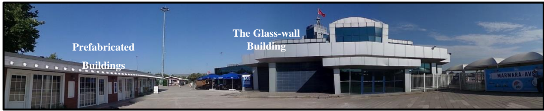
Figure 19: A view of the prefabricated buildings at Yenikapı.
