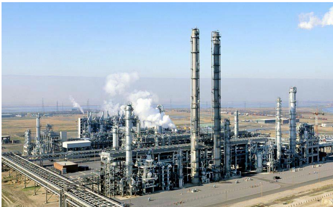
Figure 5.1 Steam Cracker and Fractionator (Hot& Cold) sections of the ethylene plant (Alper, 2012)
