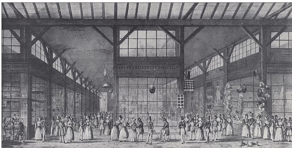
Figure 4.19. Palais Royal, Galleria de Bois, interior view.
