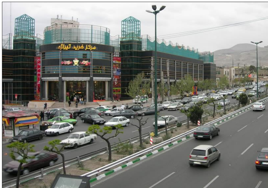
Figure 5.9. Tirajhe Shopping Mall in Tehran.
