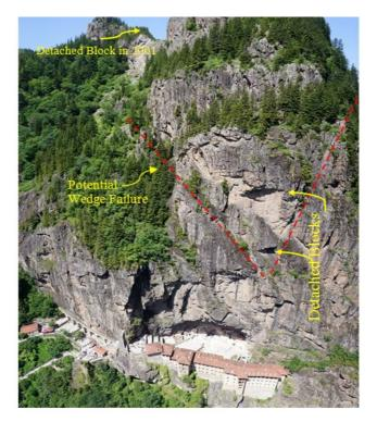
Figure 4.5 –Potential wedge failure and detached blocks from it.
