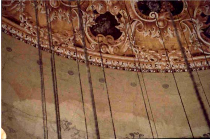
Figure 3.7. Openings for resonators within the dome of Süleymaniye Mosque (Source: Acar, 2000: 112)
