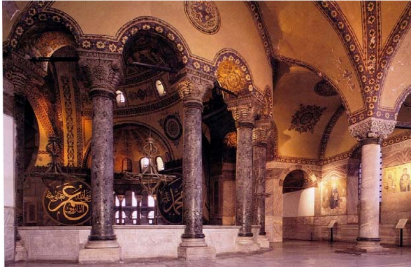
Figure 3.15. Interior view from south gallery, Hagia Sophia (Source: Akgündüz et. al, 2006: p.91)
