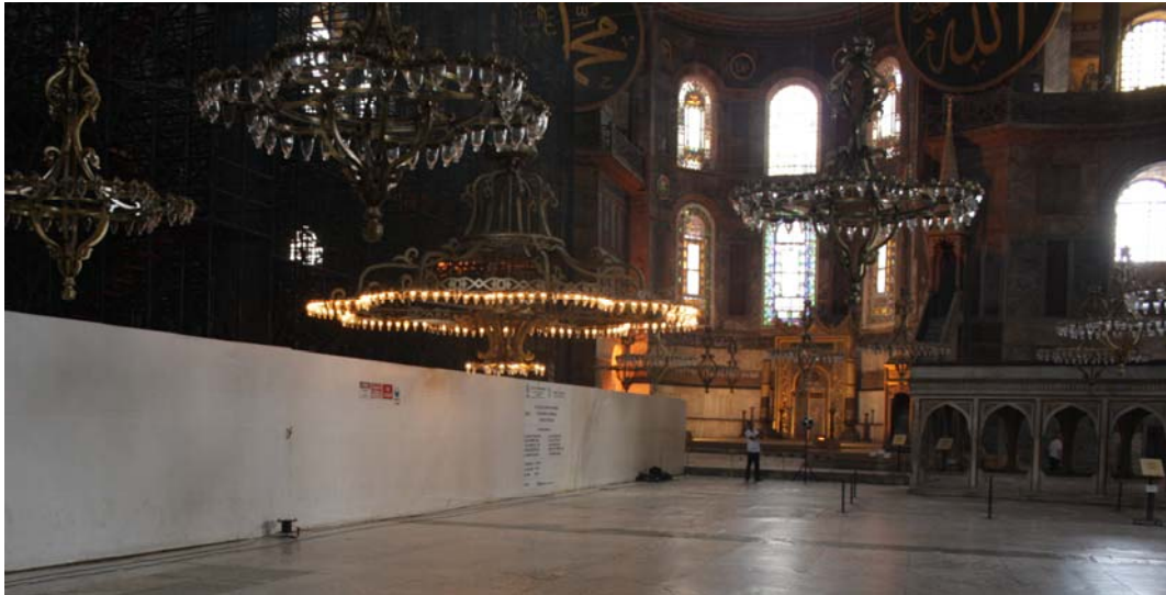
Figure 6.20. Barrier wall separating left aisle from the main space, for providing security zone in ongoing 2014 restorations, Hagia Sophia ( Source: photographed by the author )
