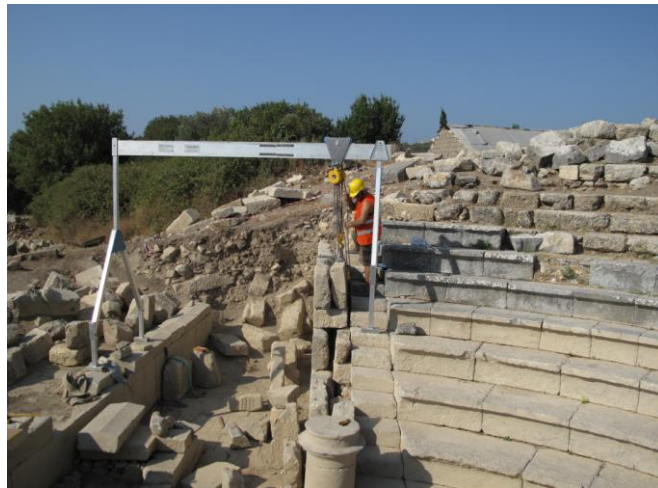
Figure 47: Anastylosis carried on the south analemma wall 214
