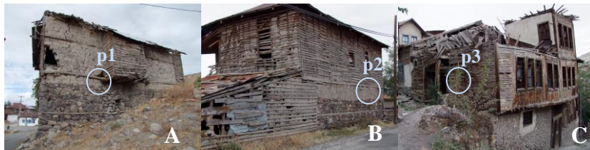
Figure 3.36 The locations where the material samples were taken from the traditional timber frame houses (A) and (B): in the village of Kavaközü with the door numbers 15 and 39 respectively; (C) in Beypazarı.
