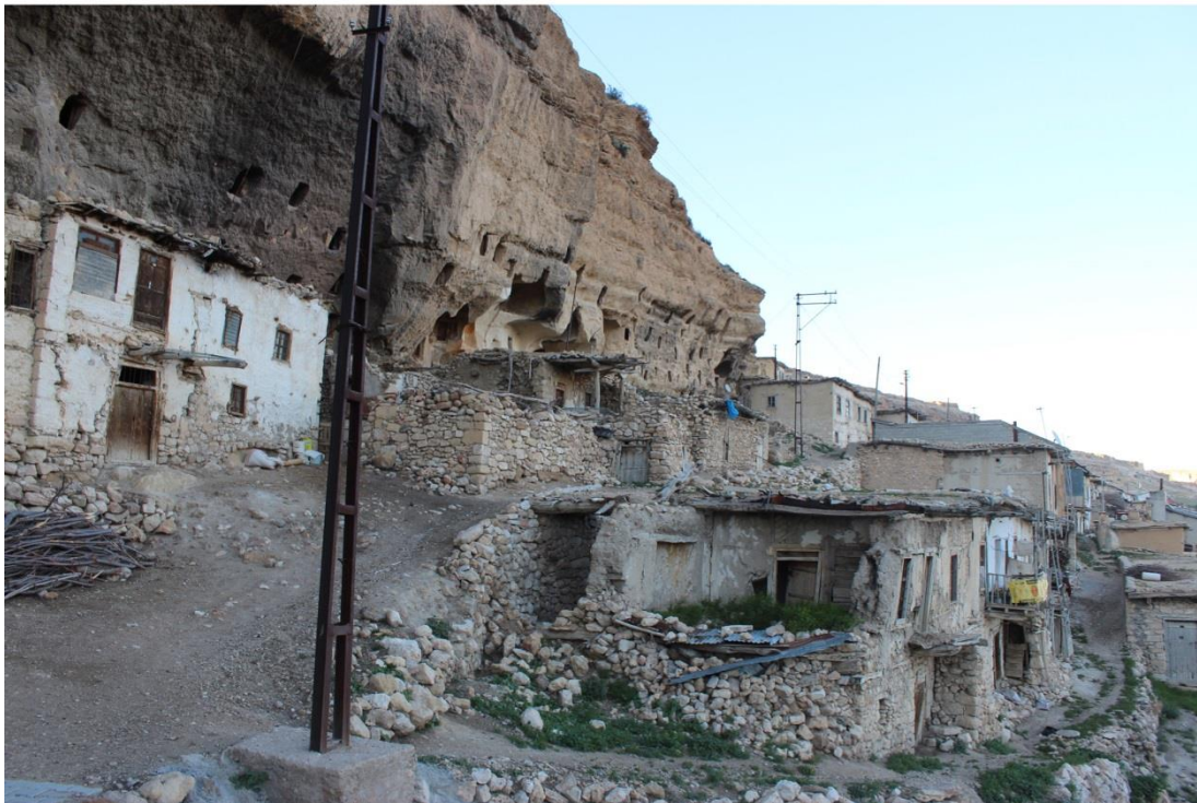
Figure 73: The demolition of the rock-cut houses and granaries 'attached' to the nature due to the Disaster Area declaration (author, May 2014)
