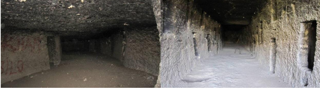
Figure 30: The rooms opening to square in 'Kum Kale' floor (left) and the square of ' At Meydanı ' floor (right) (Manazan Caves Conservation Plan notes)
