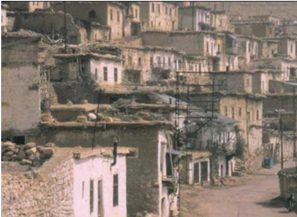
Figure 57: House Type 3: Terraced houses, the plan and section of the terraced houses (Özkan, 1992), the terraced houses (Taşkale Municipality Archive)
