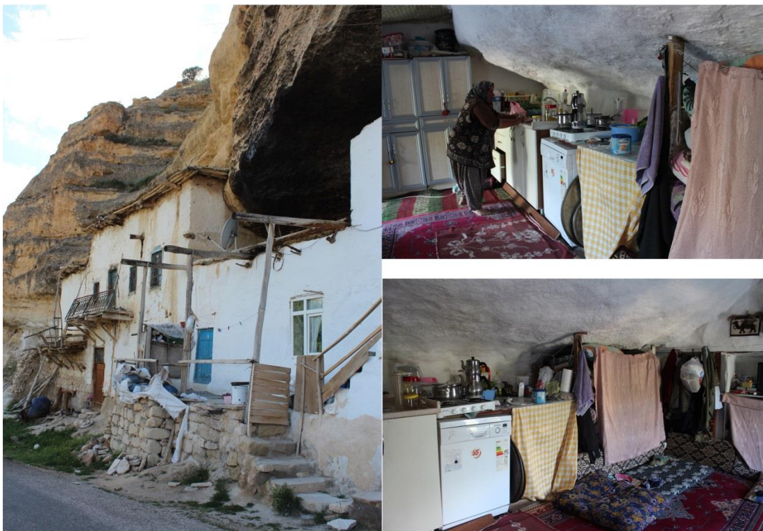
Figure 55: House Type 1: Rock-Cut Houses, 1a: Totally carved, only the front façade is built by stone masonry (top) (author, May 2014), 1b: Half-carved, half built (bottom) (author, May 2014)
