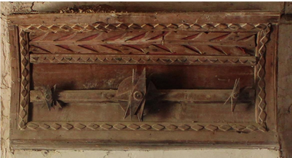
Figure 61: The inside of a traditional house, the ornamentations and the use of color, the red fabric put inbetween two layers of wooden element (author, May 2014)
