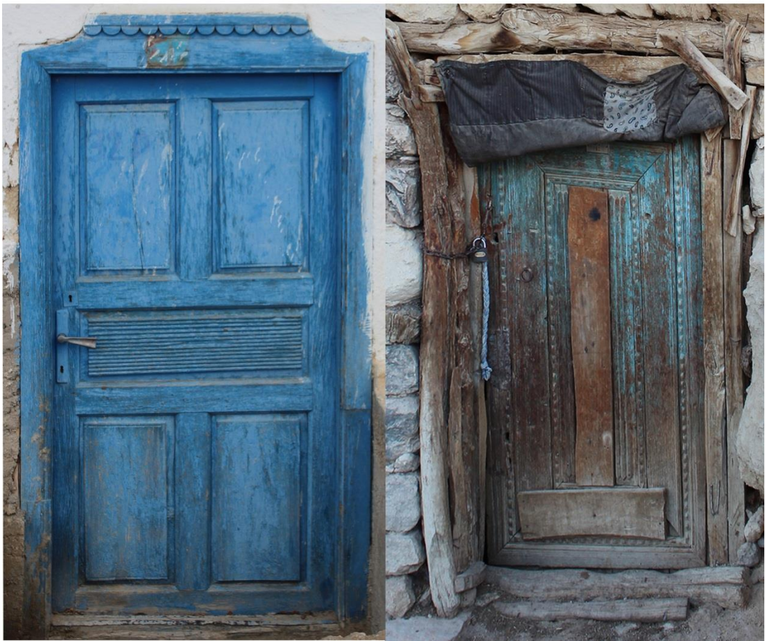
Figure 60: The exterior doors of the traditional houses (author, May 2014)
